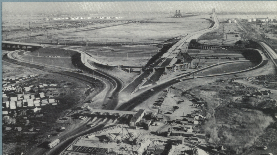
Looking east at Newark Bay-Hudson County extension from Newark Airport area
