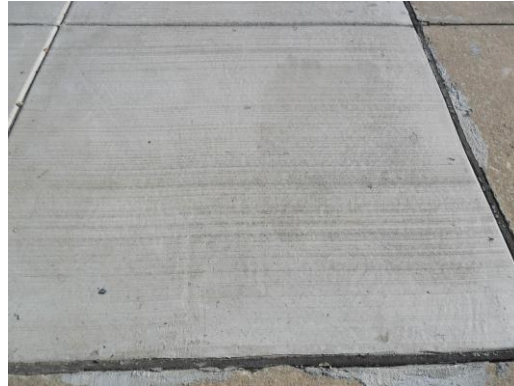
Figure 10. Pavement replacement near Wilson Hall condition on August 9, 2012. The figure on the left is a section using a RCA mix and the section on the right is a companion section that used natural aggregate
