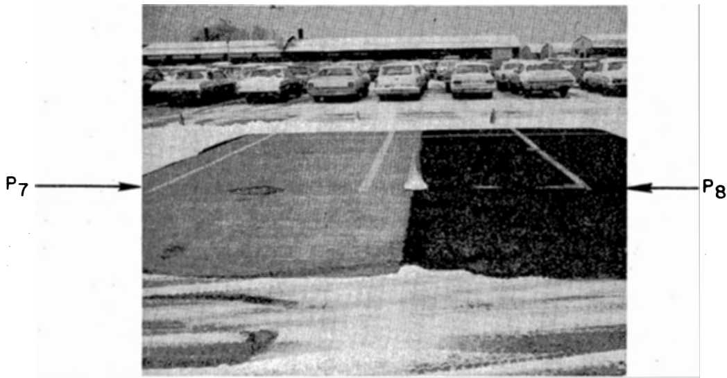
PHOTOGRAPH D-8 STORM #3 Panel #7 (Portland Cement Concrete) and Panel #8 (Bituminous Concrete) 9:00 AM - February 7, 1972 (16 hours from turn-on)(Air Temp. 29.3°F)
