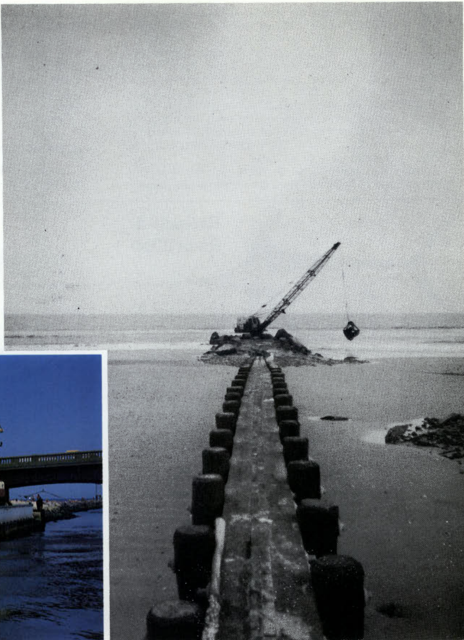
▲ Rebuilding a Stone Groin, Strathmere
