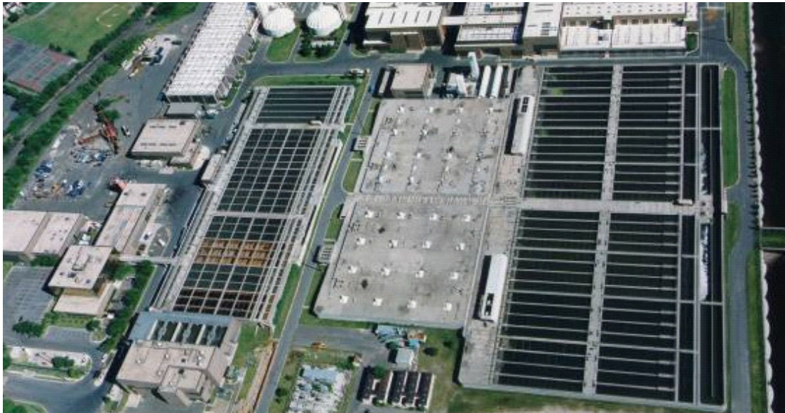
Above is pictured the CCMUA's facility featuring improvements as issued through NJEIPF loans.
