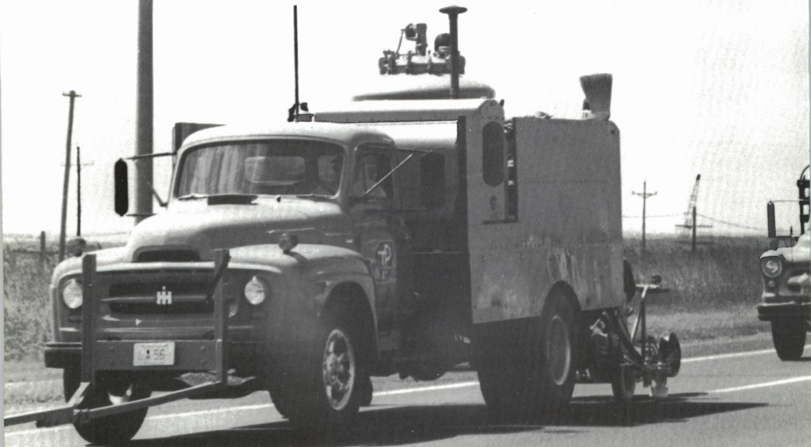
Turnpike line striping machine in operation
