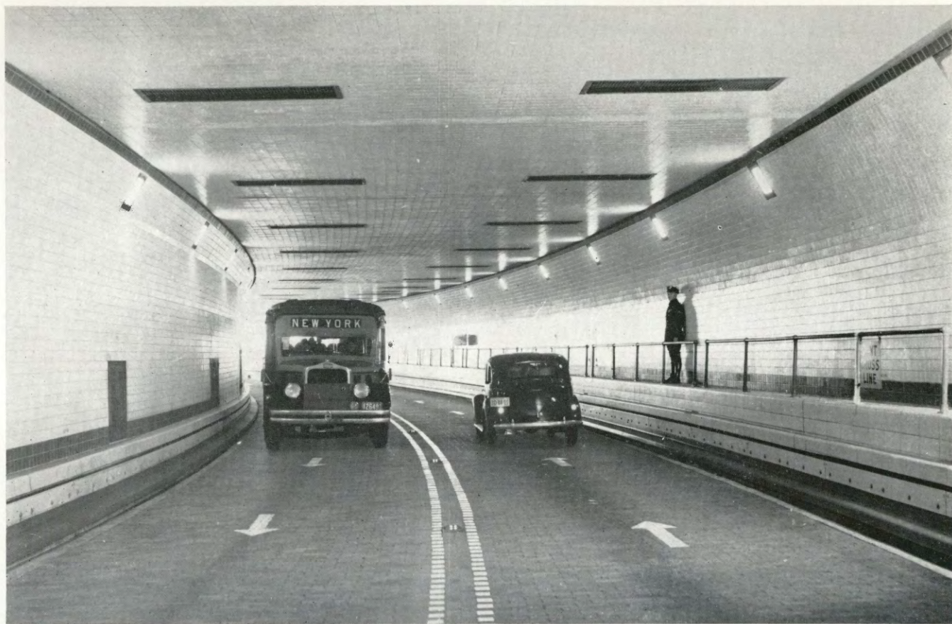
Lincoln Tunnel — First Operating Unit — Interior
