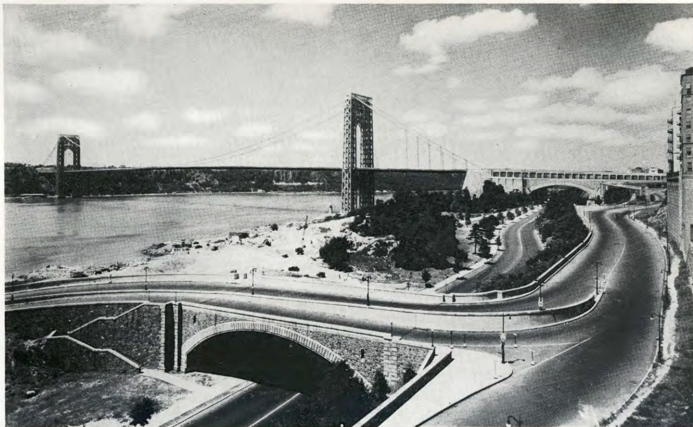
George Washington Bridge — Proposed Finish for Anchorage and Arch over Riverside Drive
