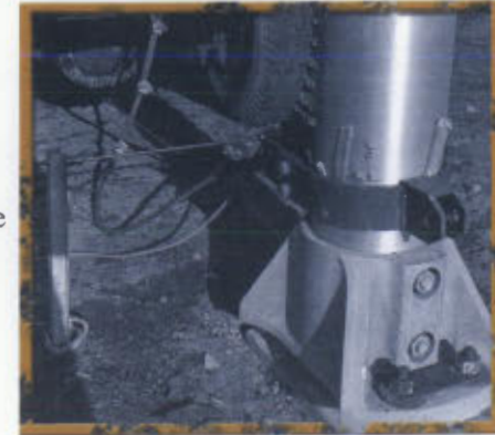
NJ breakaway signs, a national first, lessen impacts on drivers in accidents thanks to this load concentrated breakaway coupling.
