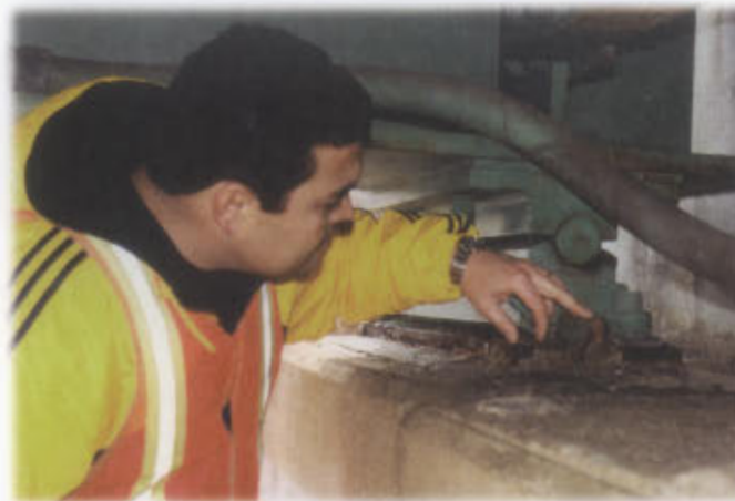
Assistant Engineer Mujahid Khan evaluates the bearing rocker of the Interstate I-195 South Broad Street bridge in Trenton.
