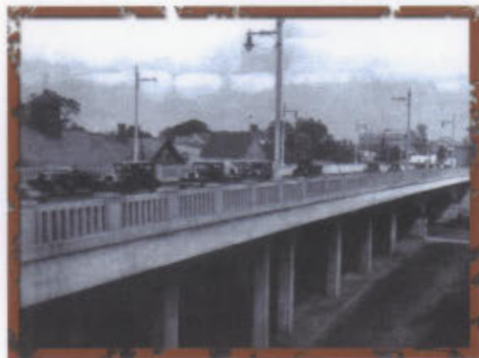
The 1929 Elizabeth River viaduct bridge’s original construction was 55 feet wide; the new bridge will have a 108-foot width.
