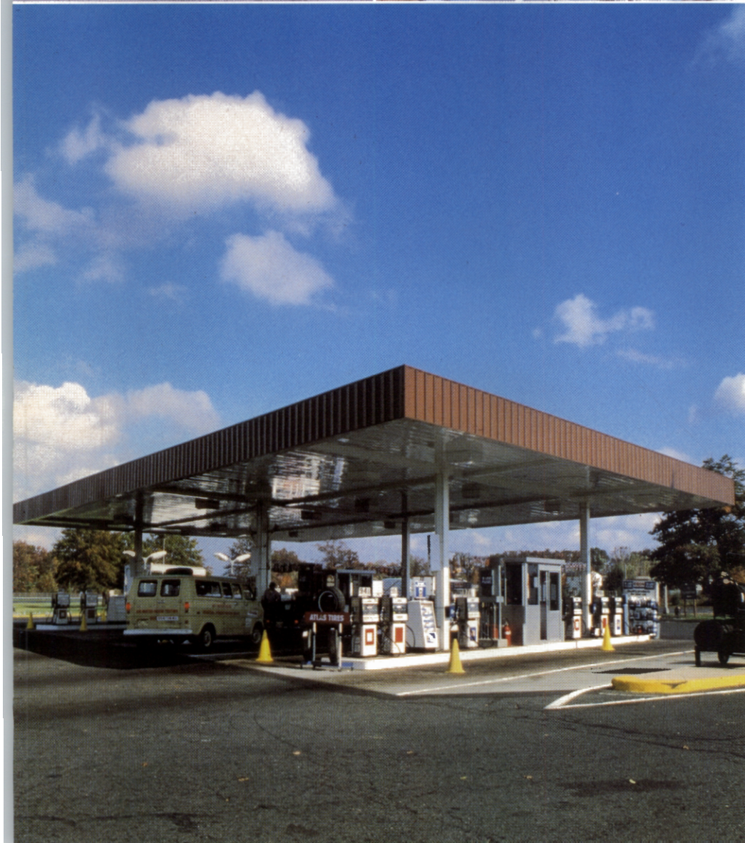
Pump islands at the Joyce Kilmer Service Area blossom forth with a new protective canopy to make dispensing of fuel more convenient.
