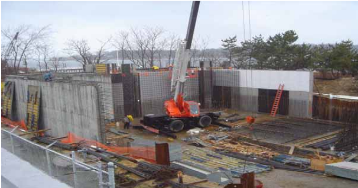
CONSTRUCTION OF SBR BASIN Photo Courtesy of Steve Hearl, CH2M, PC
