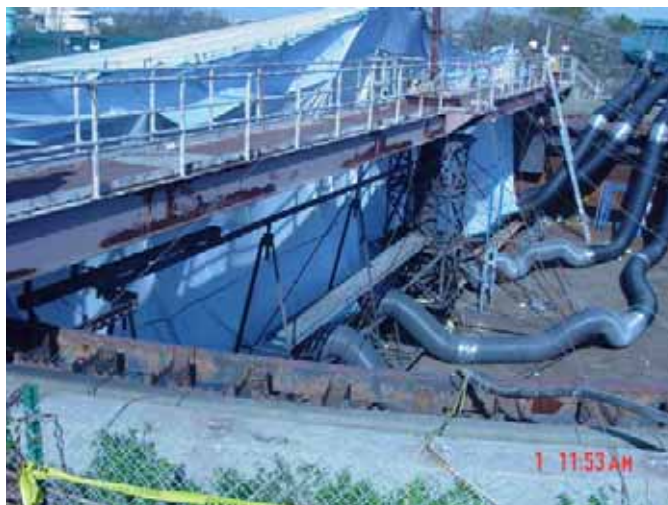
FINAL TANK REFURBISHING Photo Courtesy of Suffolk County DPW
