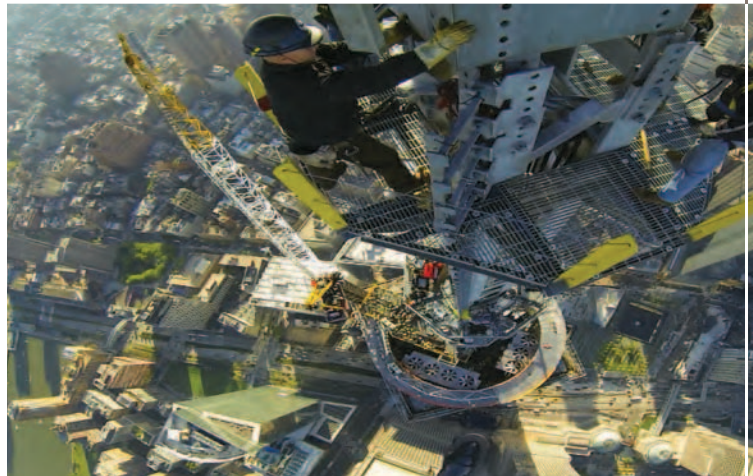
Installing the final section of the spire atop One WTC
