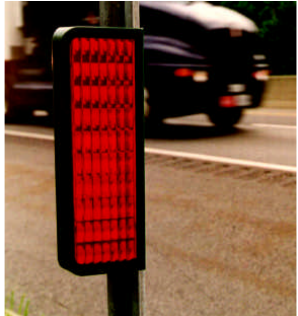
Low intensity reflected light from vehicle headlights is directed from the road onto the roadside area to discourage deer from attempting to cross the road.
