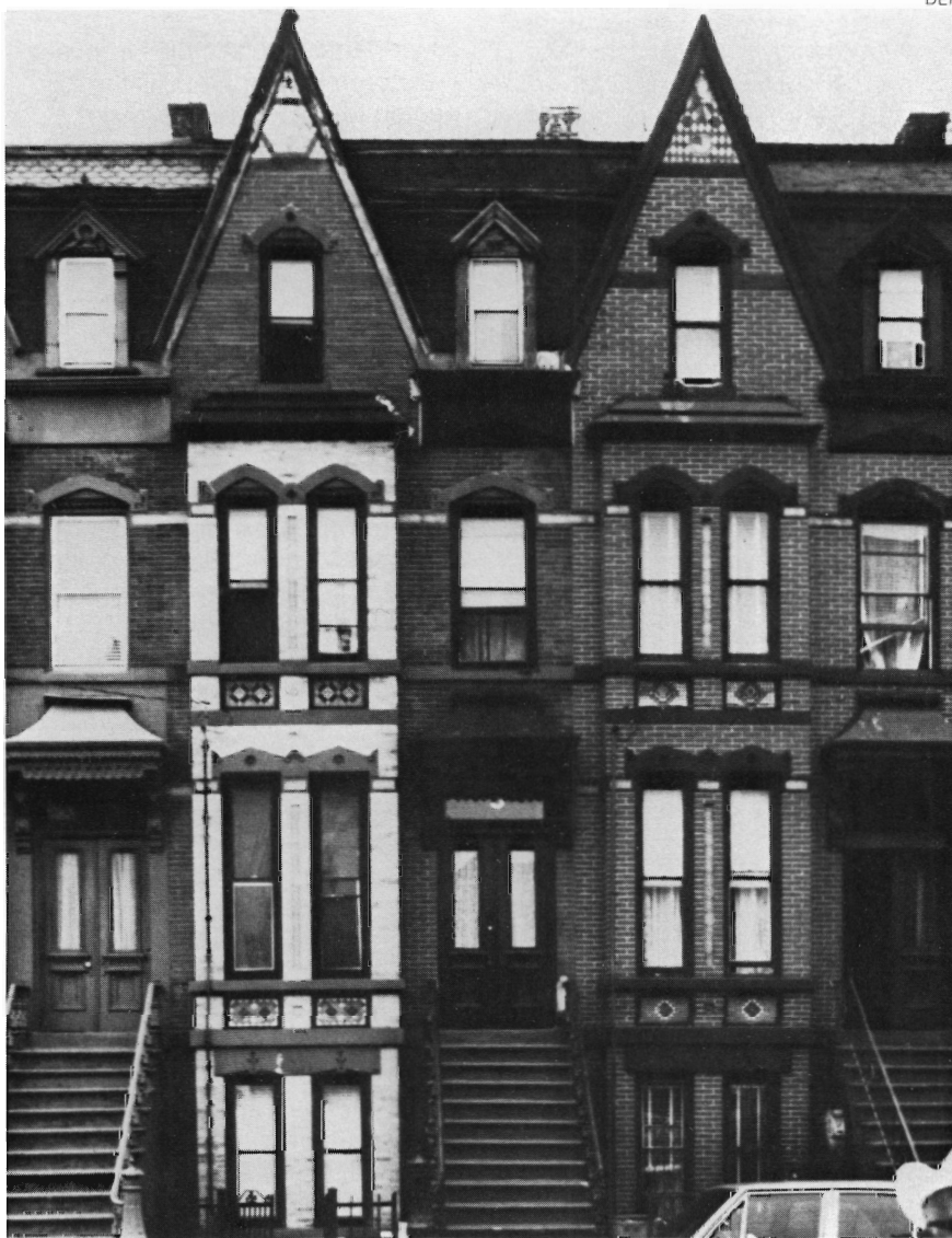
These distinctive late 19th Century rowhouses were listed on the National Register in 1980 as part of the Van Vorst Historic District in Jersey City.
