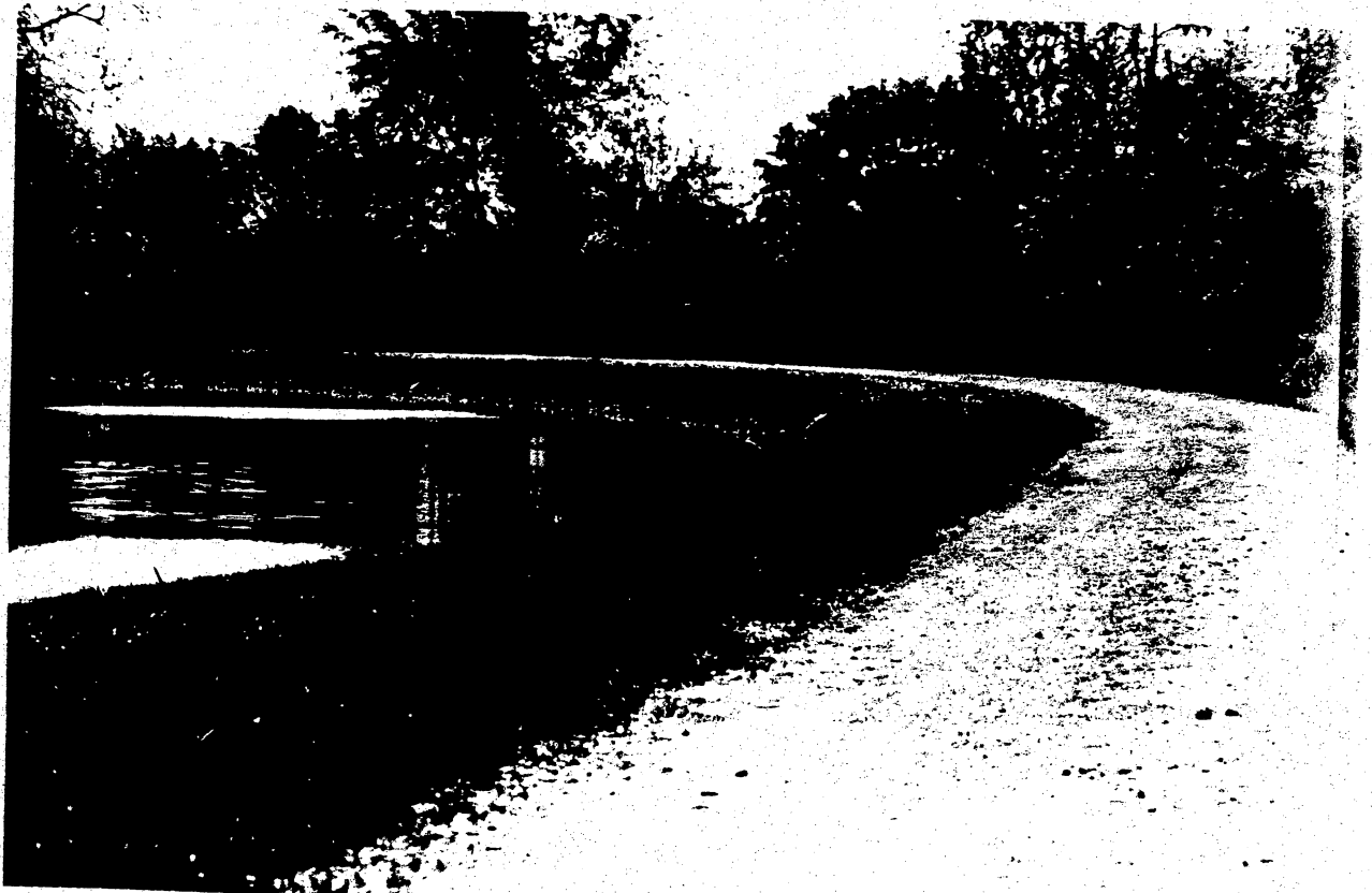
Two more views of the towpath of the feeder canal near Lambertville, looking downstream. Top picture: coarse crushed stone on embankment and towpath. Bottom: grass on embankment, fine crushed stone on towpath.
