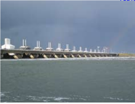
The Eastern Scheldt Barrier protects residents of the Netherlands's Zeeland Province from North Sea storm surges. The barrier consists of gates that are only closed during extreme high tides allowing water to continue to flow through the tidal inlet. (Photo by Amy Shallcross)
