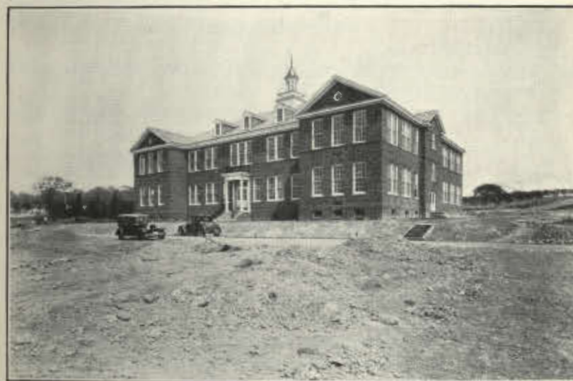
The School Building Nearing Completion
