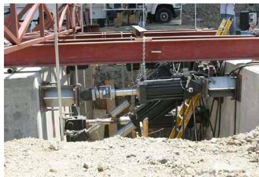
Figure IV.B.2 Photograph of actuator configuration
