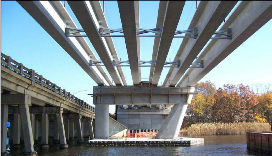
Figure 5.99 Route 70 Over Manasquan River Bridge during construction
