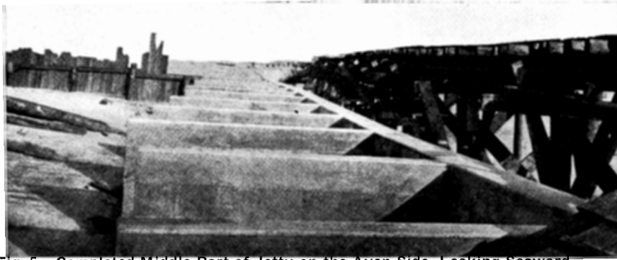
Fig. 5. Completed Middle Part of Jetty on the Avon Side, Looking Seaward. Railroad Trestle Will be Removed.
