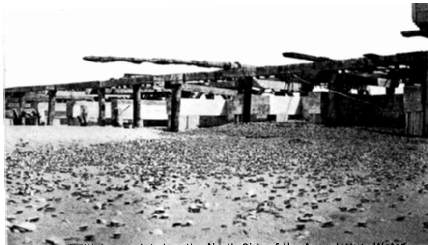
Fig. 6. Sand Fill Accumulated on the North Side of the Avon Jetty; Water was 6-10 Feet Deep Here When Jetty was Built.
