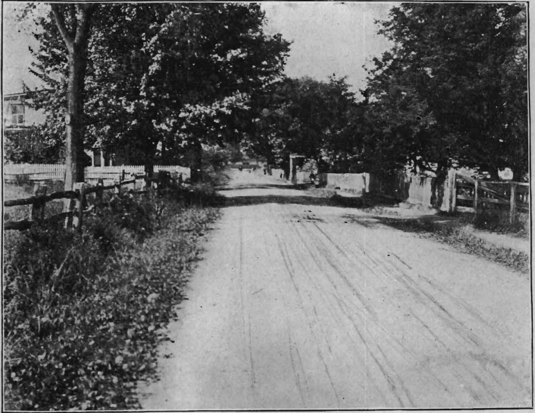
Lodi, N. J., Bergen Co. Four-inch Macadam Pavement carrying heavy traffic.
