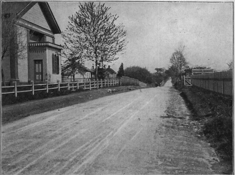
Union St., Lodi, N. J., Bergen Co. Four-inch Macadam, carries a heavy brick and ice traffic—150 loads per day of 3 to 5 tons on narrow tires. W. C. Foster, Engineer.
