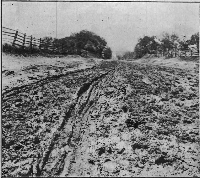
Kaighn's Ave. Extension, Camden Co., N. J. Before.
