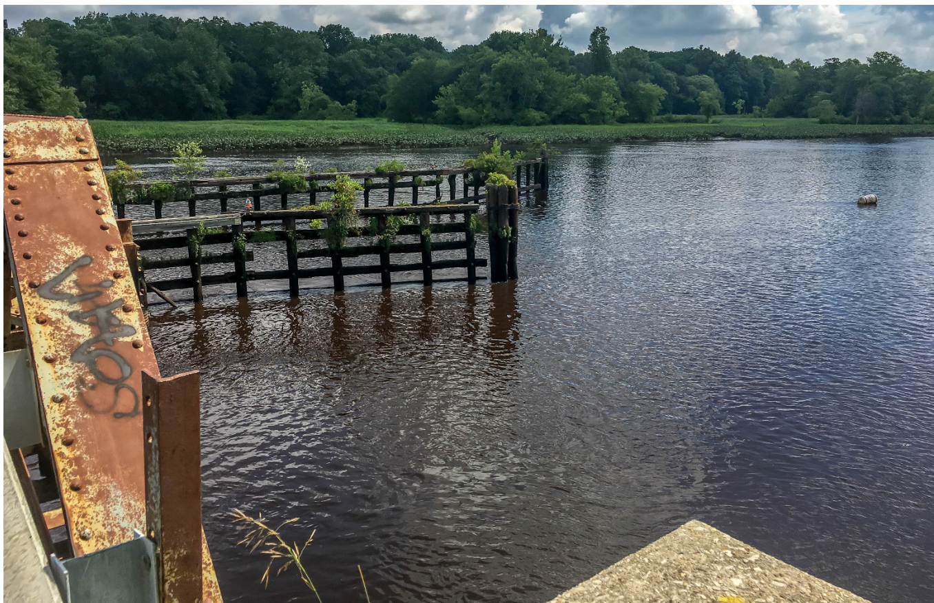
Centerton Road Bridge Demolition, Burlington County
