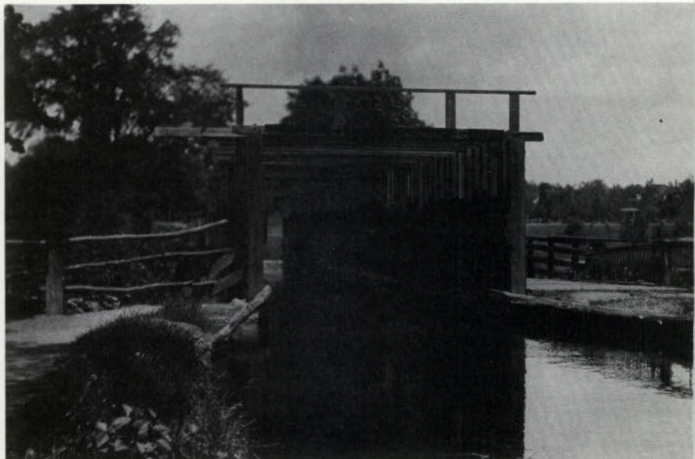
Aqueduct over Passaic River at Little Falls
