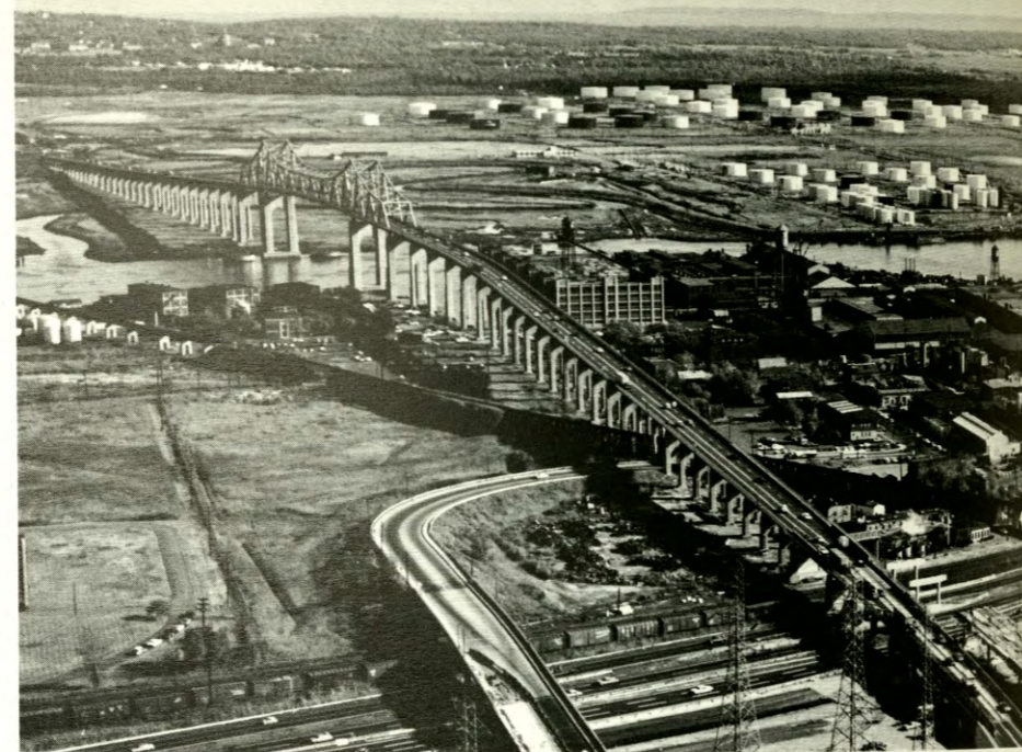
Much of the new traffic generated at the six Port Authority crossings was recorded at the three Staten Island Bridges and especially at the Goethals Bridge, (above) which experienced an exceptional 99.9 percent rise over 1964.
