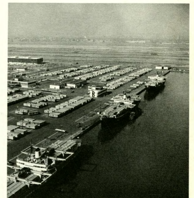
On the cover: The vast 703-acre Elizabeth-Port Authority Marine Terminal is being developed with facilities specifically planned to handle containerized cargo. Early in 1965, work started on the erection of four dockside mobile gantry cranes which will be used by Sea-Land Service, Inc.
