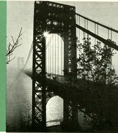
Tunnels and Bridges 48
