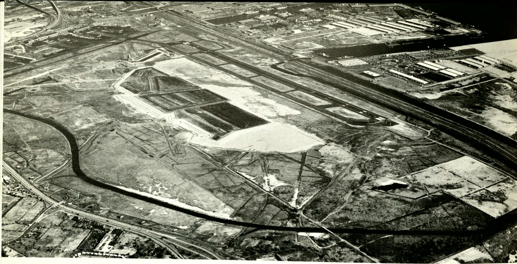
Site preparation for the new Newark Airport terminal complex progressed with the placement of over 14,000,000 cubic yards of hydraulic fill and surcharge on a 450-acre area in the center of the airfield.
