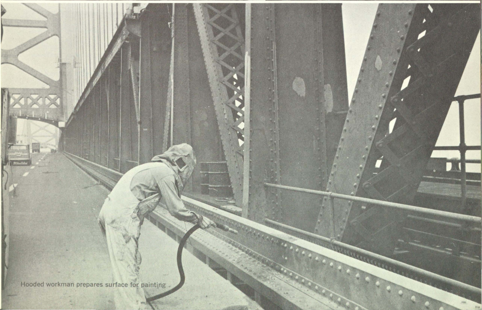
Painters aloft on bridge
