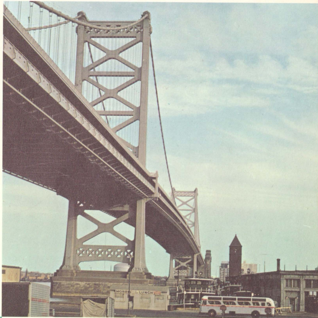
Benjamin Franklin Bridge, from Race Street, Philadelphia
