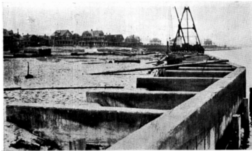
Fig. 5. The Finished Portion of the South Jetty and the Derrick Scow Used in Setting Piles.
