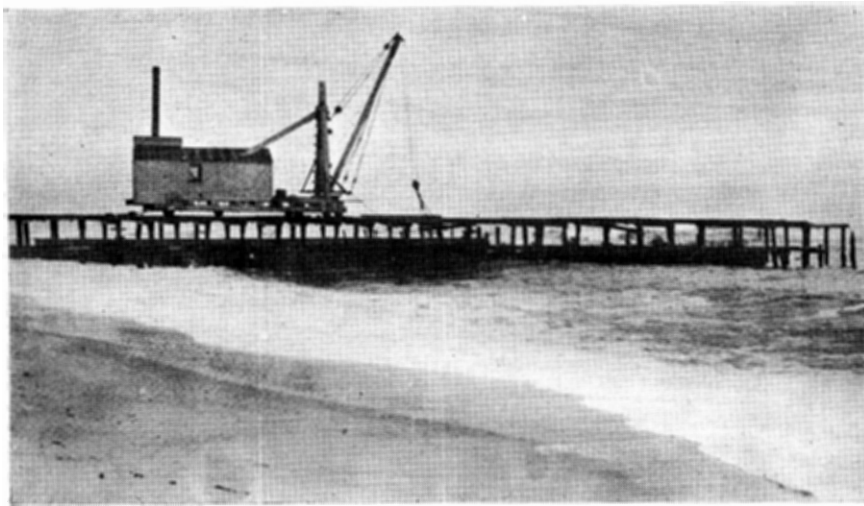
Fig. 4. A Portion of the North Jetty, With False Work and Traveling Crane. The Seaward End of the False Work and Some of the Concrete Piles Were Swept Away by the Storms of Last Winter.
