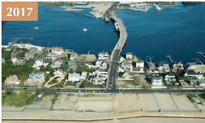
Figure 10. In 2012, Superstorm Sandy breached the barrier island at Mantoloking Bridge and Route 35, joining the ocean and the bay and destroying houses. Over the course of the last 5 years, the recovery has moved slowly. Other coastal communities with strong beach and dune complexes tended to have much less damage.
