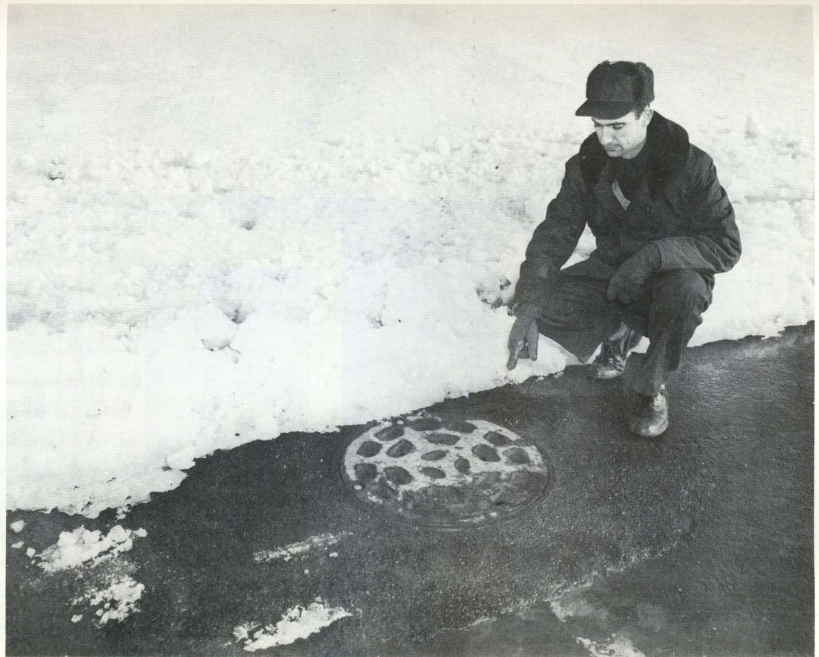
NEWLY INSTALLED CATCH BASIN.
