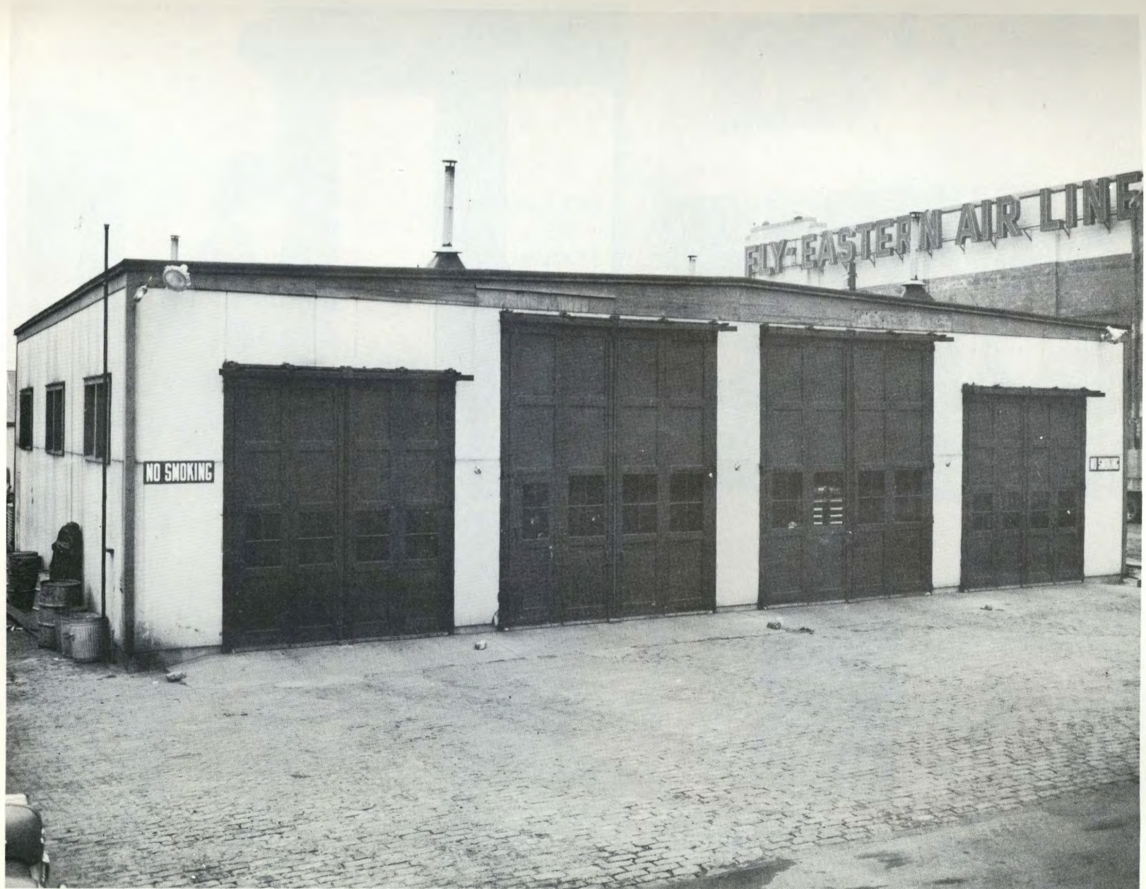
NEW EMERGENCY DOORS ON TEMPORARY GARAGE.
