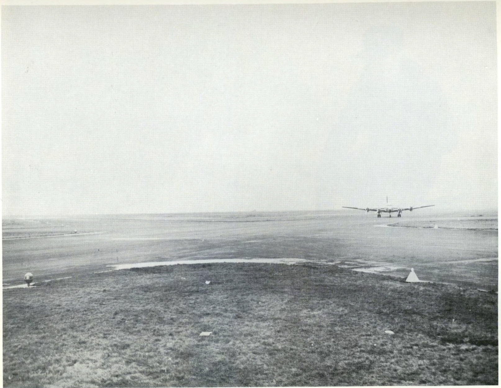
ELEVATED CONE-TYPE LIGHTS, RUNWAY 1-19.
