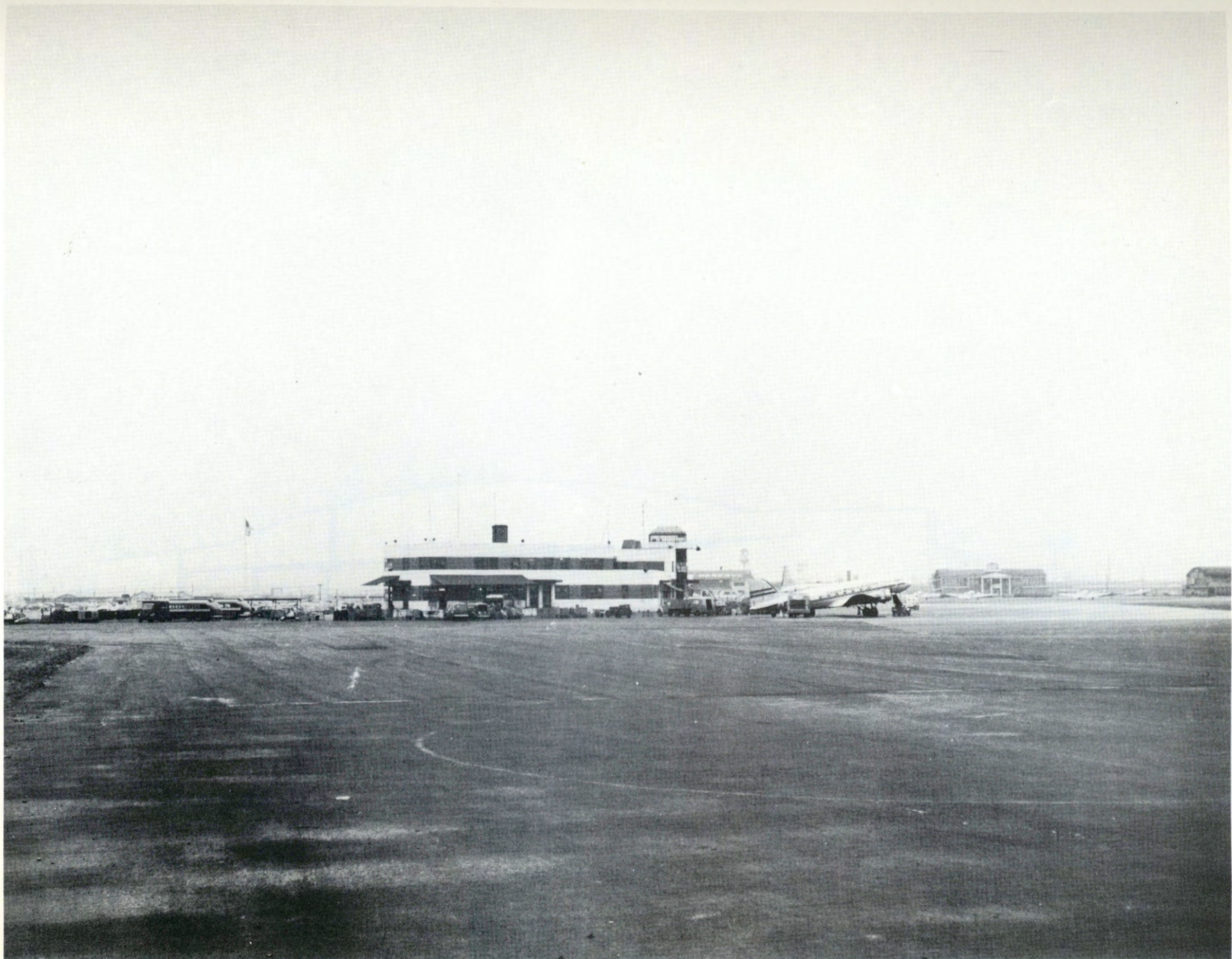
NEW PAVEMENT ON RUNWAY NEAR ADMINISTRATION BUILDING.
