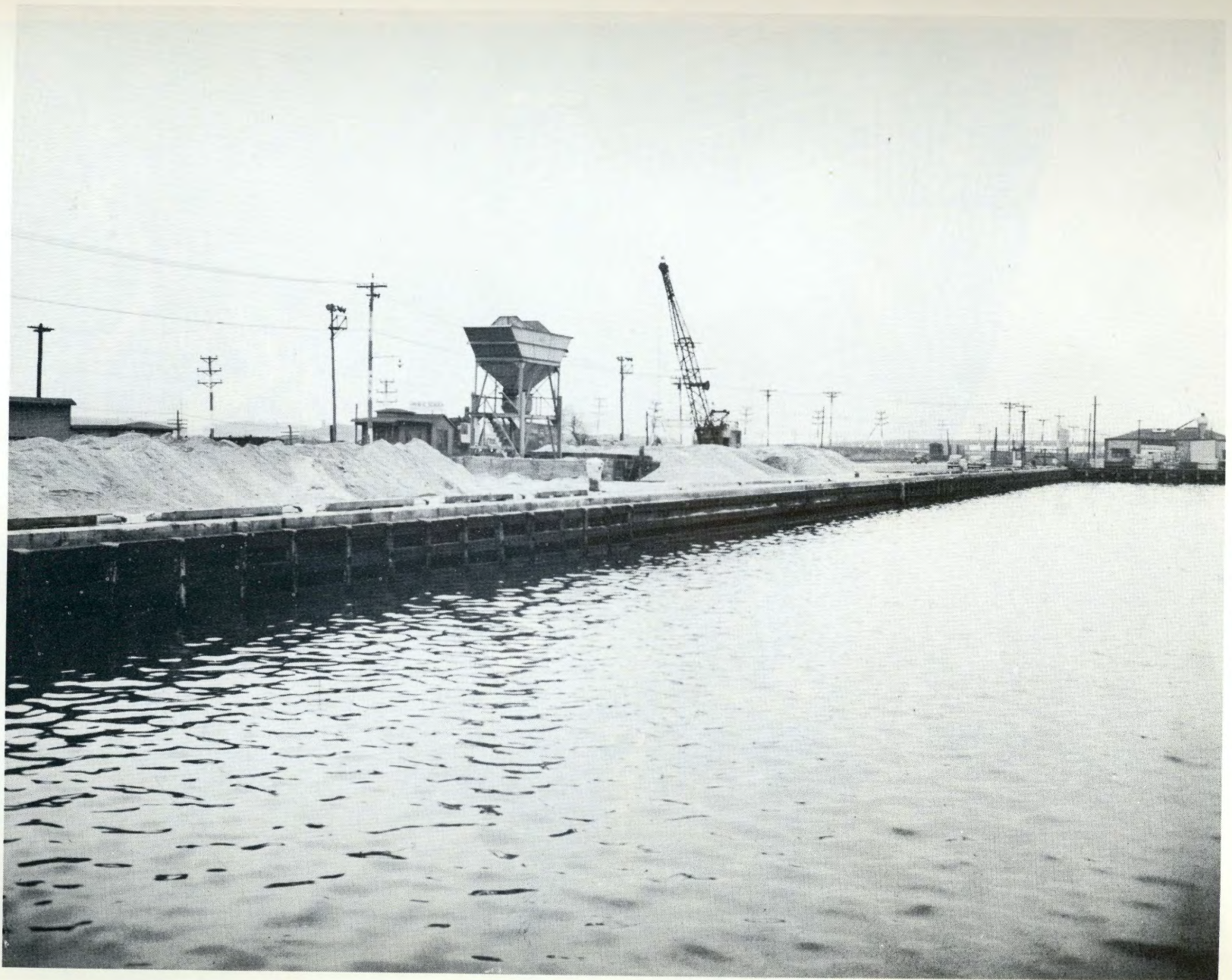
HEAD OF CHANNEL, 75 PER CENT OF RECONSTRUCTION OF FENDER SYSTEM COMPLETED.
