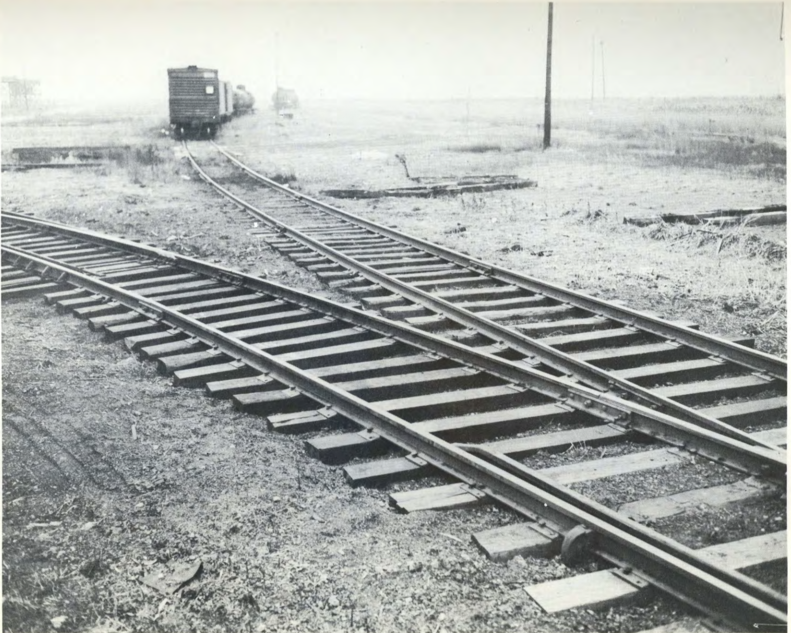
INTERNAL RAILROAD TRACK SYSTEM - REHABILITATION COMPLETED.
