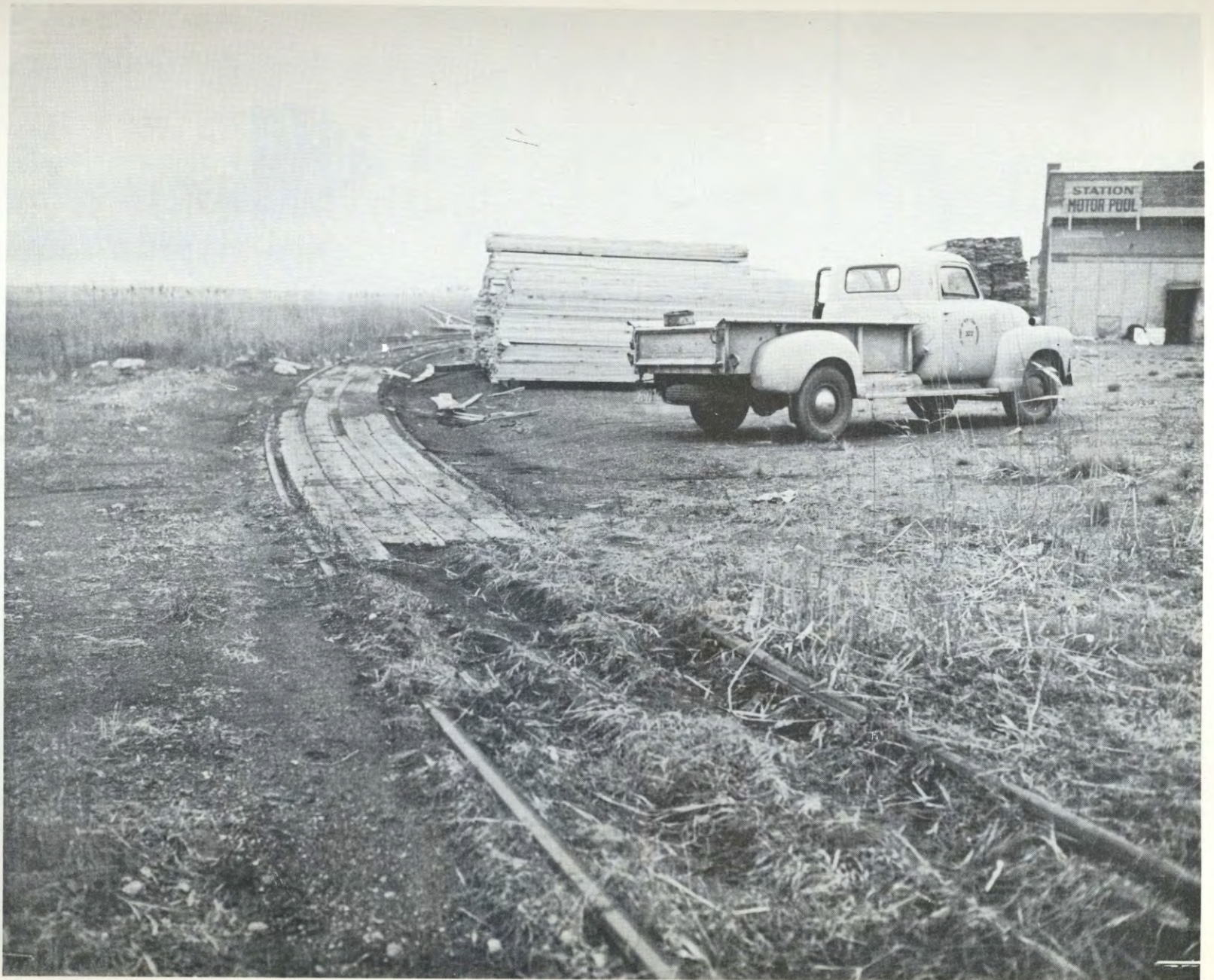
INTERNAL RAILROAD TRACK SYSTEM - TRACKS COVERED BY DEBRIS.
