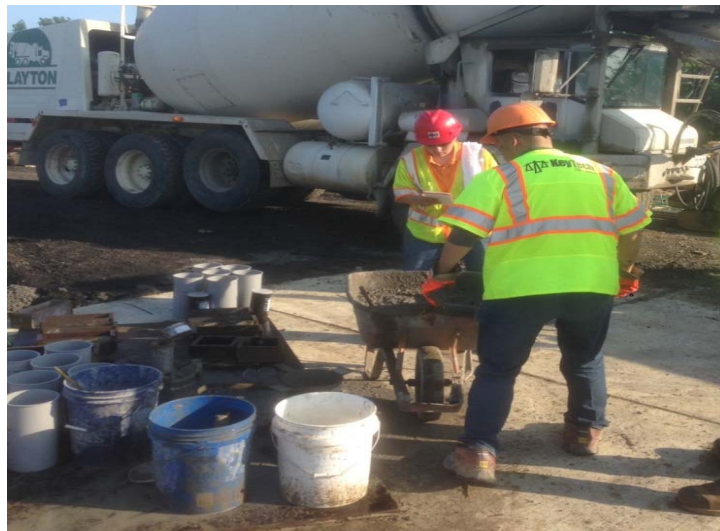
Figure 12. Quality Control Professionals Transporting Fresh Concrete for Slump and Air Pressure Testing
