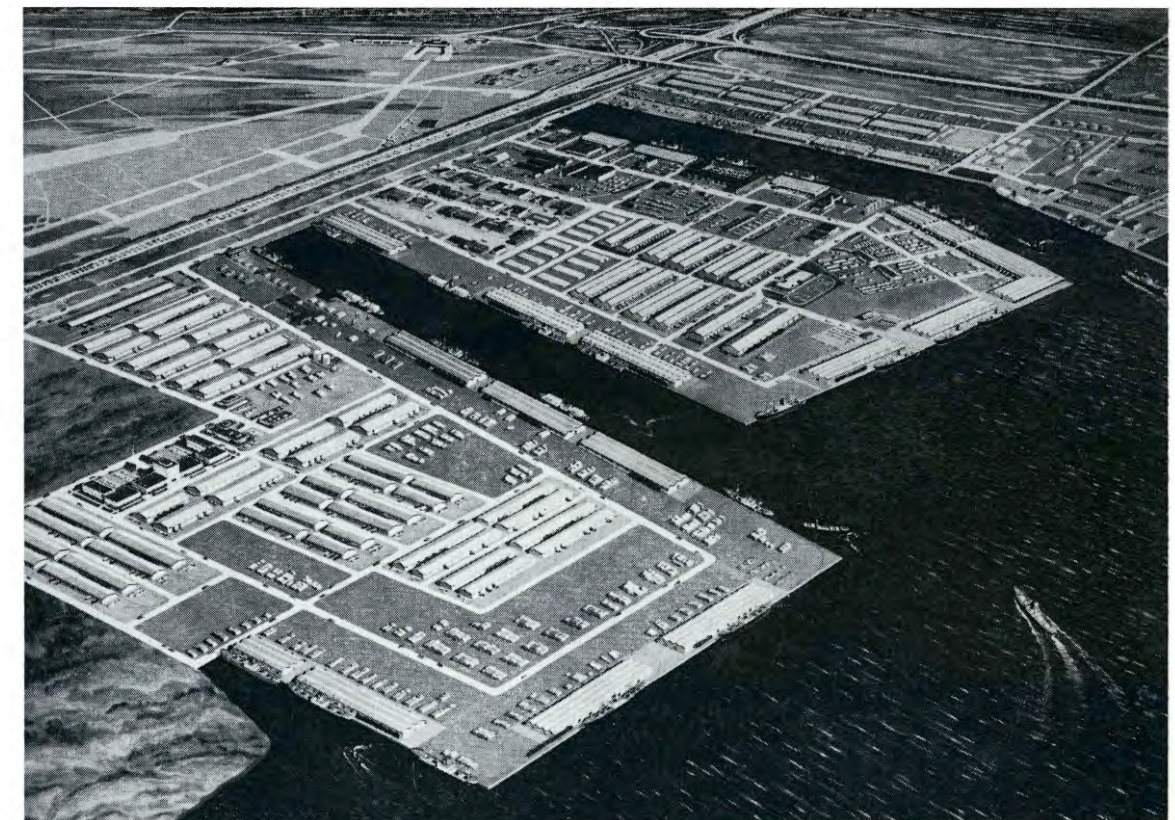
Artist's rendering of Port Newark and the Elizabeth-Port Authority Piers shows the two marine terminals as they will appear upon completion of development. They will handle 11,000,000 tons of cargo a year at 62 deep-water vessel berths.
