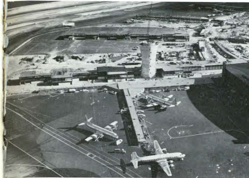
Construction of a new runway, control tower, and finger buildings of the Central Terminal Building as part of the LaGuardia Airport redevelopment program was carried out with service to 3,293,000 commercial passengers in 1961.
