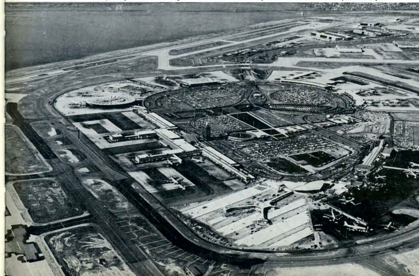
New York International Airport, the second busiest air terminal in the nation for air carrier movements, served 10,147,000 commercial air passengers in 1961 and 226,000 aircraft movements. Construction of two individual passenger terminal buildings in the 655-acre Terminal City advanced toward their completion this year.
