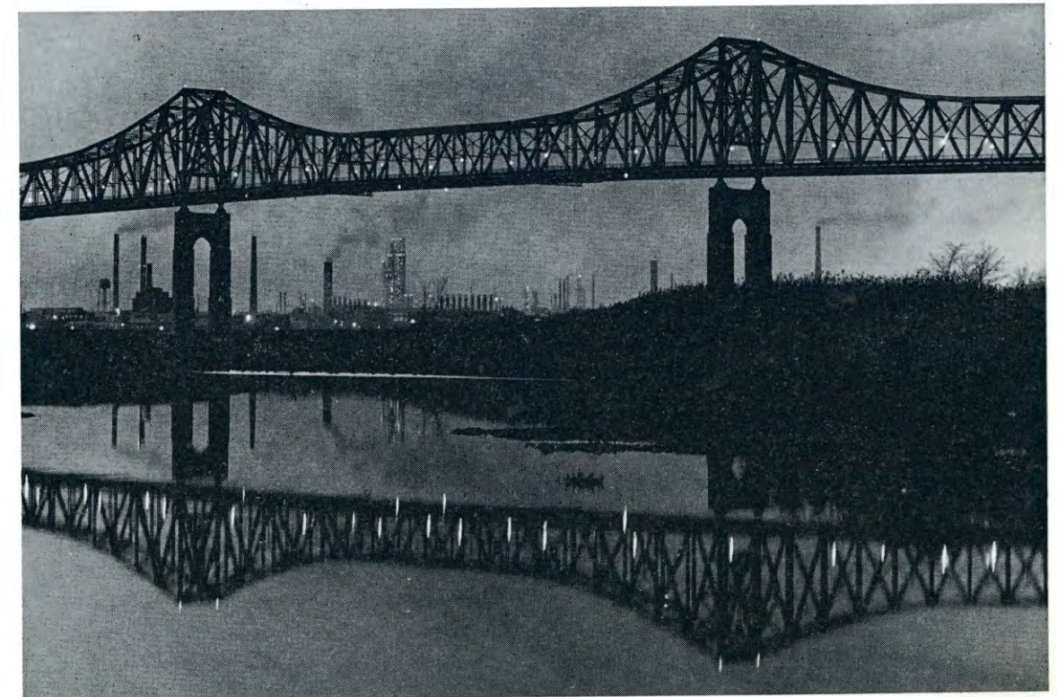
The Outerbridge Crossing linking Staten Island with Perth Amboy, New Jersey, was opened to traffic in 1928. The Bridge is undergoing an extensive rehabilitation and improvement program to serve future traffic needs.
