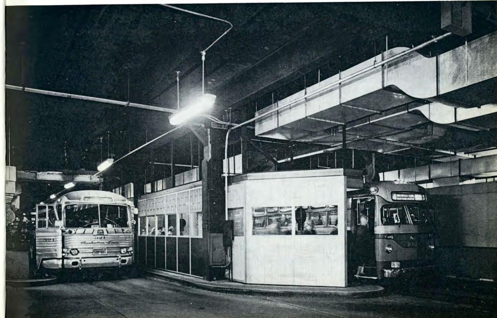
Ventilation improvements on bus operating platforms throughout the busy terminal are an integral part of the Bus Terminal expansion program. Shown above is an enclosed and ventilated platform on the Suburban Bus Level.
