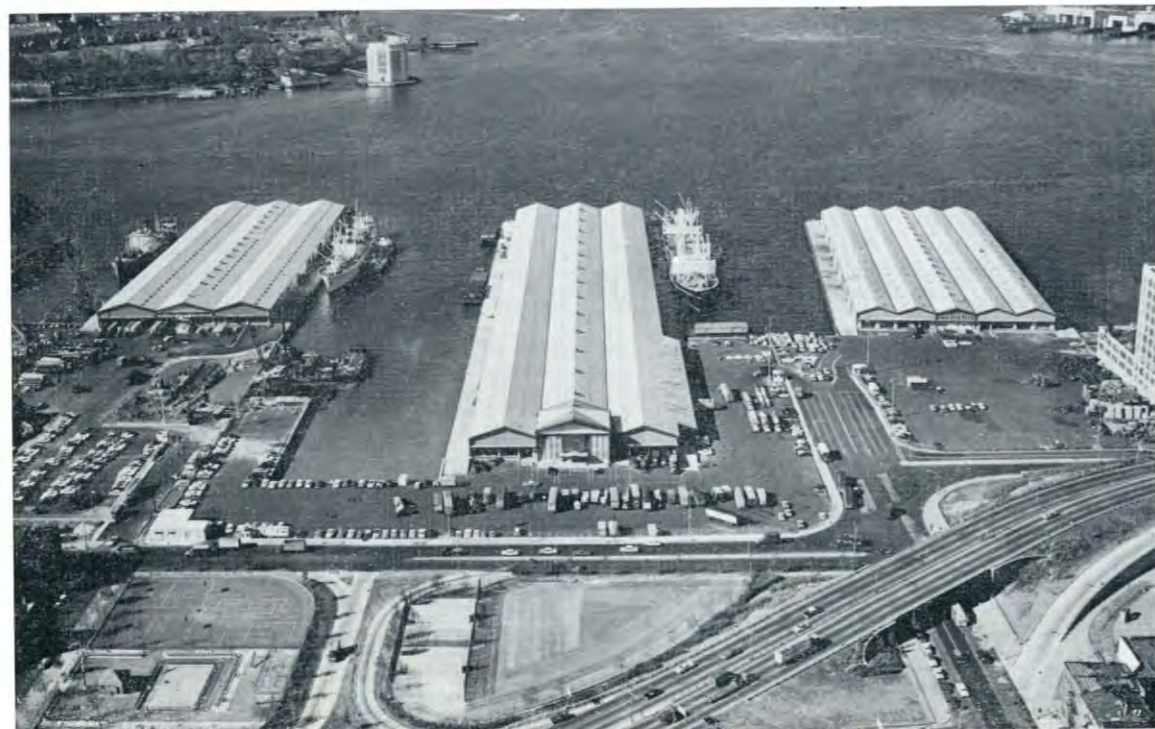
New Piers 6 (right), 7, and 8 (left) in the Baltic Terminal Area of the Brooklyn-Port Authority Piers were completed and put into operation during 1961. Eight of the thirteen new piers called for are serving the maritime industry.
