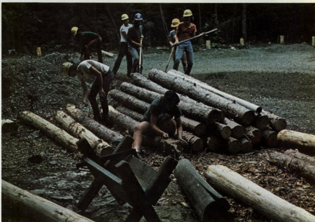
Above: Stokes Forest YCC'ers enclose one of the many areas they have worked on in the forest. This parking lot uses timbers cut from Stokes' many Red Pine plantations and its groves of Black Locust. Top right: A beautiful stone retaining wall is built at Stoney Lake in Stokes Forest. The stone is found in the forest and even the concrete blocks are recycled. Below: An excellent example of using natural materials to be found in the forest. A YCC'er's notches a Red Pine log for a fence crosspiece.
