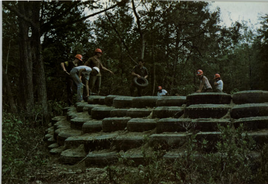
Above: Superintendent Louis Cherepy works with YCC'ers placing used tires in Sunrise Mountain containing wall. Rutgers student Sandy Henricks (white hard hat) is Work Leader on the project. The terracing effect and the packing with sand can be noted in this scene. Right: The completed bridge across Stoney Brook. Some of the lumber used is new but much is recycled.
