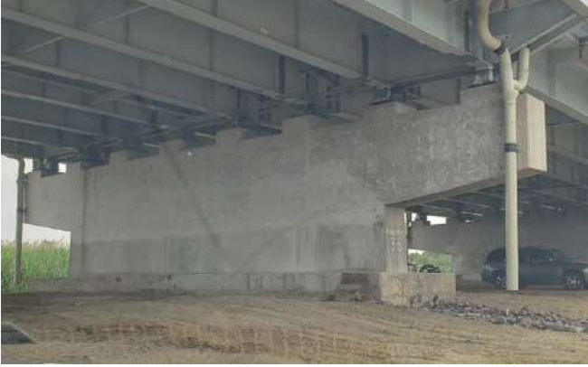
As structures age, the need for larger rehabilitation projects increase. For example, eleven concrete piers at the Commodore Barry Bridge were recently replaced.
