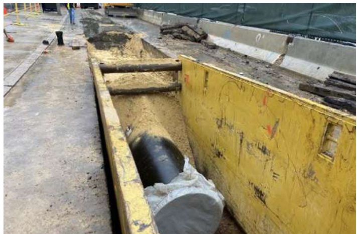
Installation of a new 36" city water main is nearing completion.
