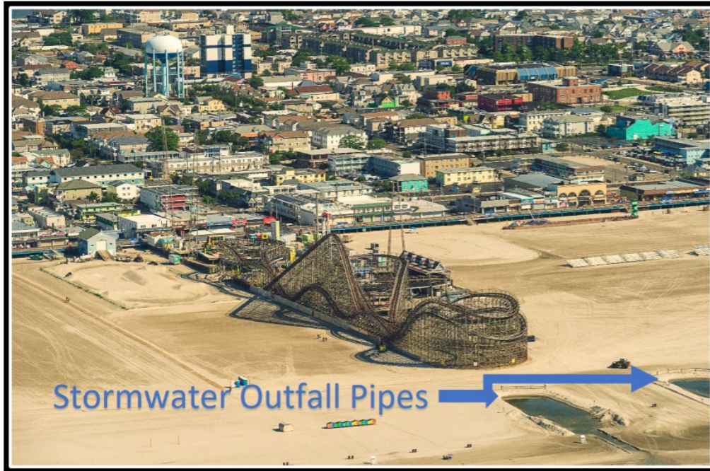
Figure 10: Stormwater Outfall Pipes in Wildwood, Cape May
