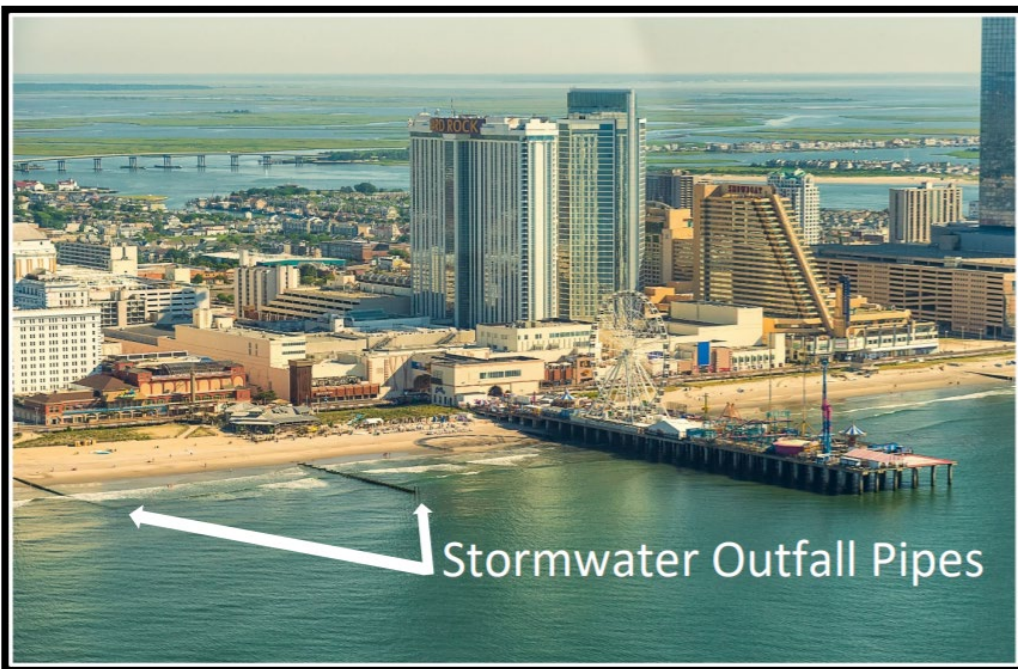
Figure 9: Stormwater Outfall Pipes in Atlantic City, Atlantic County
