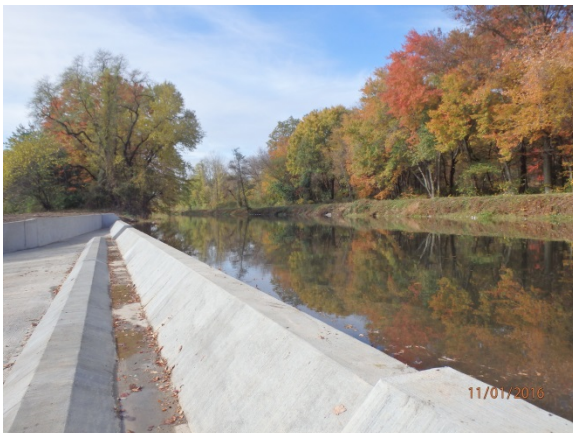
Completed Cherry Tree Lane Spillway.
