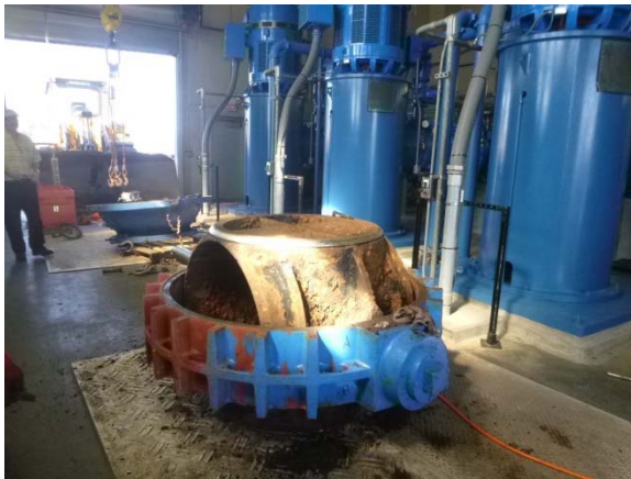
Large Valve Repair work.
