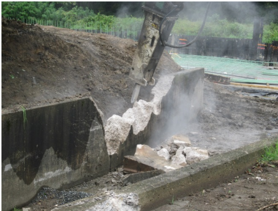
Demolition work at Cherry Tree Lane Spillway.
