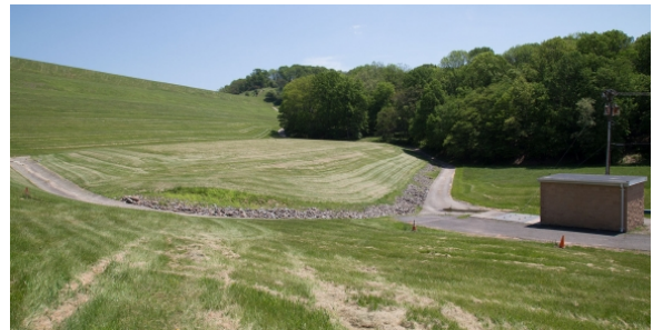
Round Valley South Dam and vault
