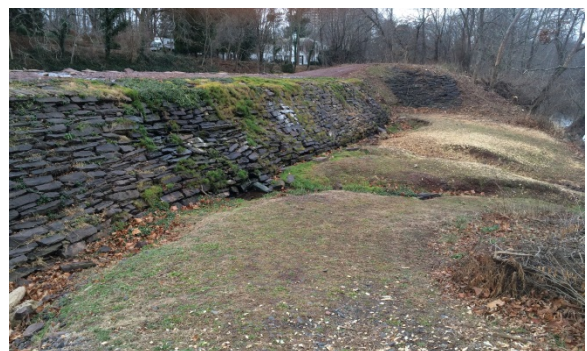
River side slope of Landing Lane Spillway.
