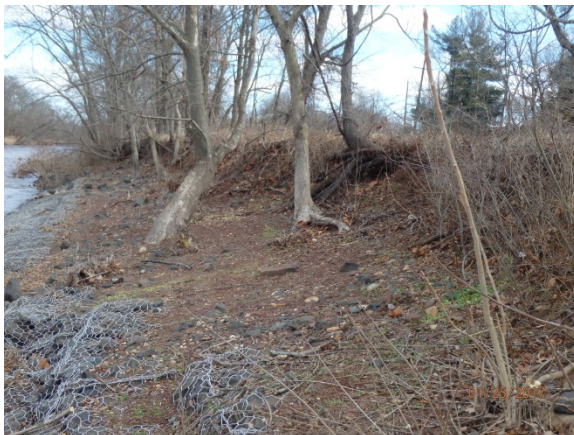
Note erosion of embankment between Raritan River (right in photo) and D&R Canal just downstream of Island Farm Weir.
