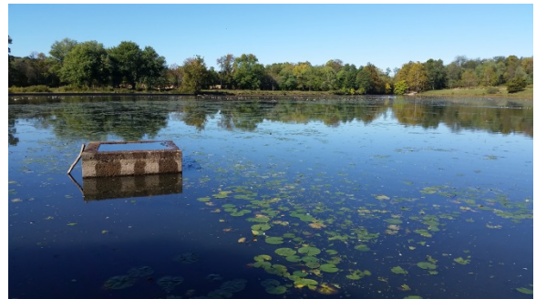
South Branch Pumping Station Intake Pond
