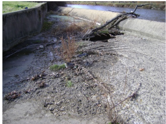
Cherry Tree Lane Spillway, before construction
