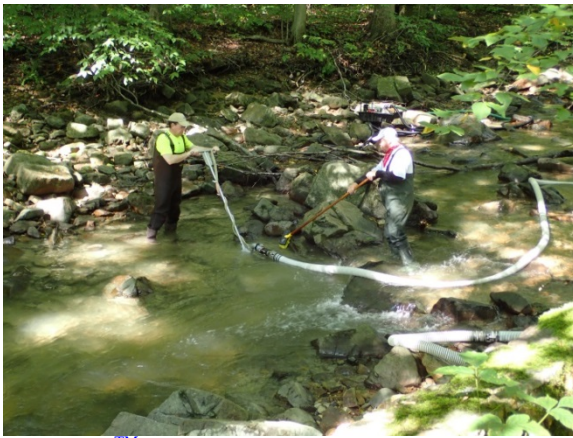
Sand Wand™ sediment removal system in use at the Spruce Run Inlet.
