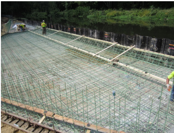
Reinforcing steel before concrete pour at Cherry Tree Lane Spillway
