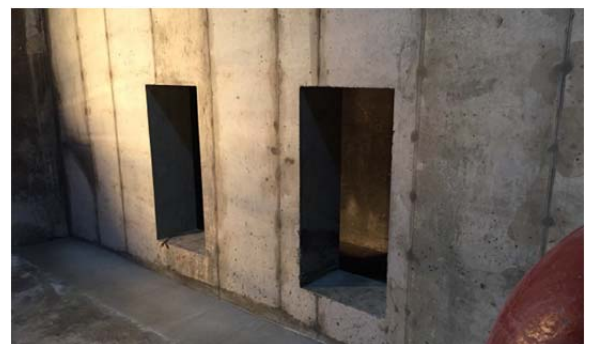
Wall and new internal piping.
