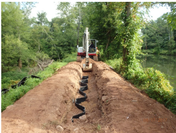
Steel sheets cut down to size will eventually be backfilled below grade. Canal to right in photo. Millstone River to the left.
