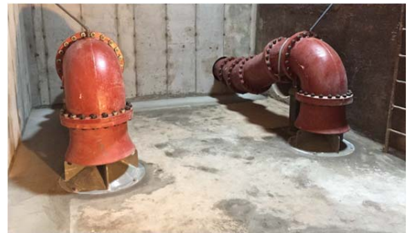
Wall and new internal piping.
