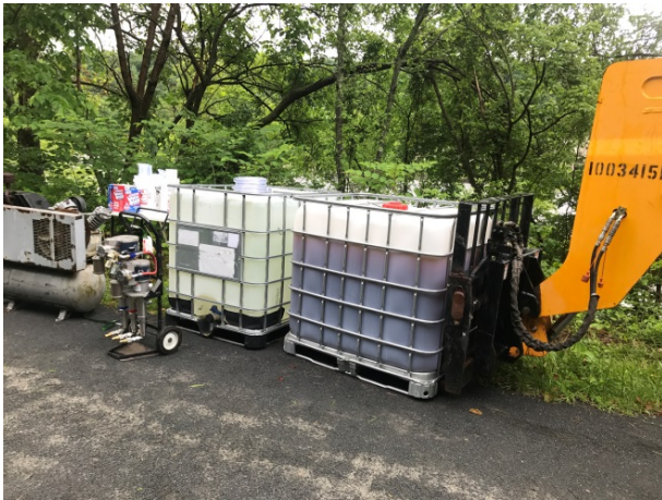
West Amwell seepage repairs. Chemical grout “totes.”
