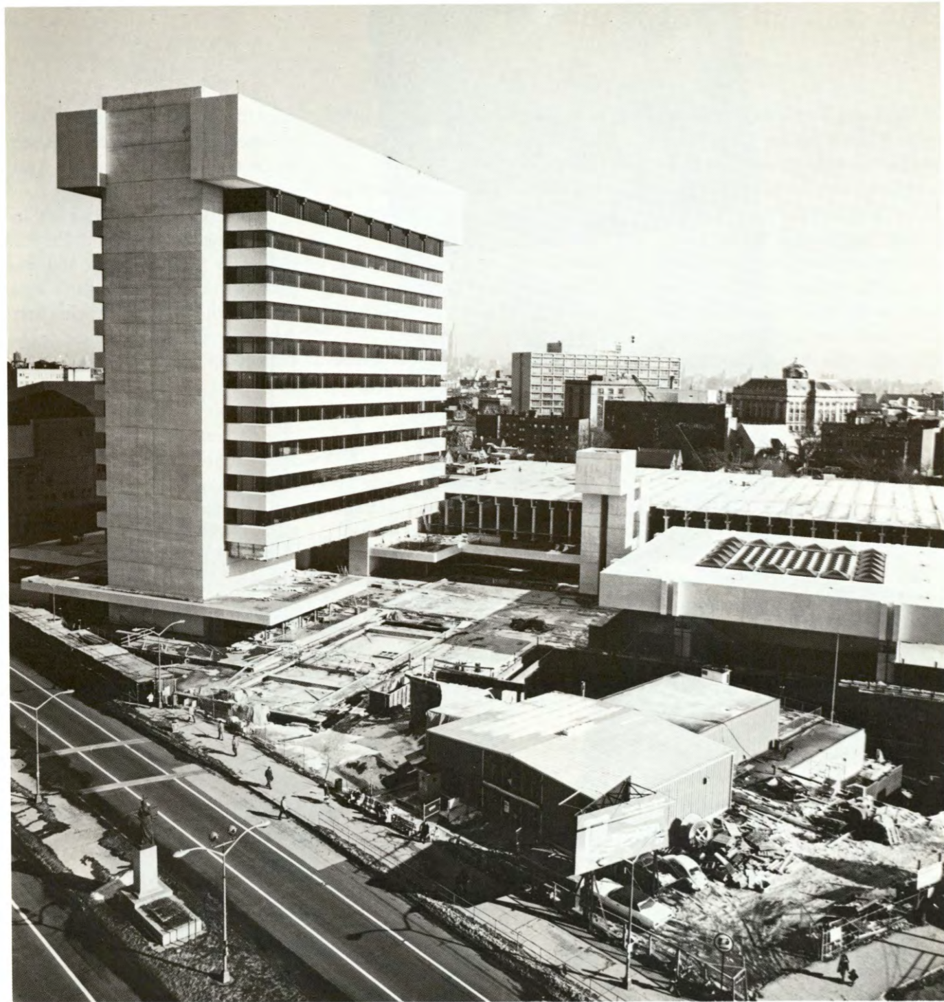
The first element of the Journal Square Transportation Center was opened in December 1973, providing the 34,000 passengers who use PATH at Journal Square daily with a new entrance with escalator service between street level and PATH platforms three levels below.
