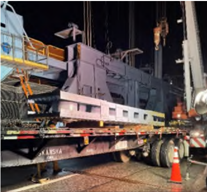
New rocker link transported to NJ Tower
