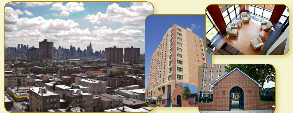
Kennedy Towers (shown above) was developed with the assistance of HMFA's Federal Low Income Housing Tax Credit Program
