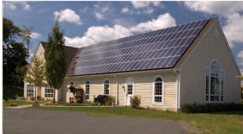
Unity Church of Sussex County installed a 16.5 kW system at no up-front cost.
