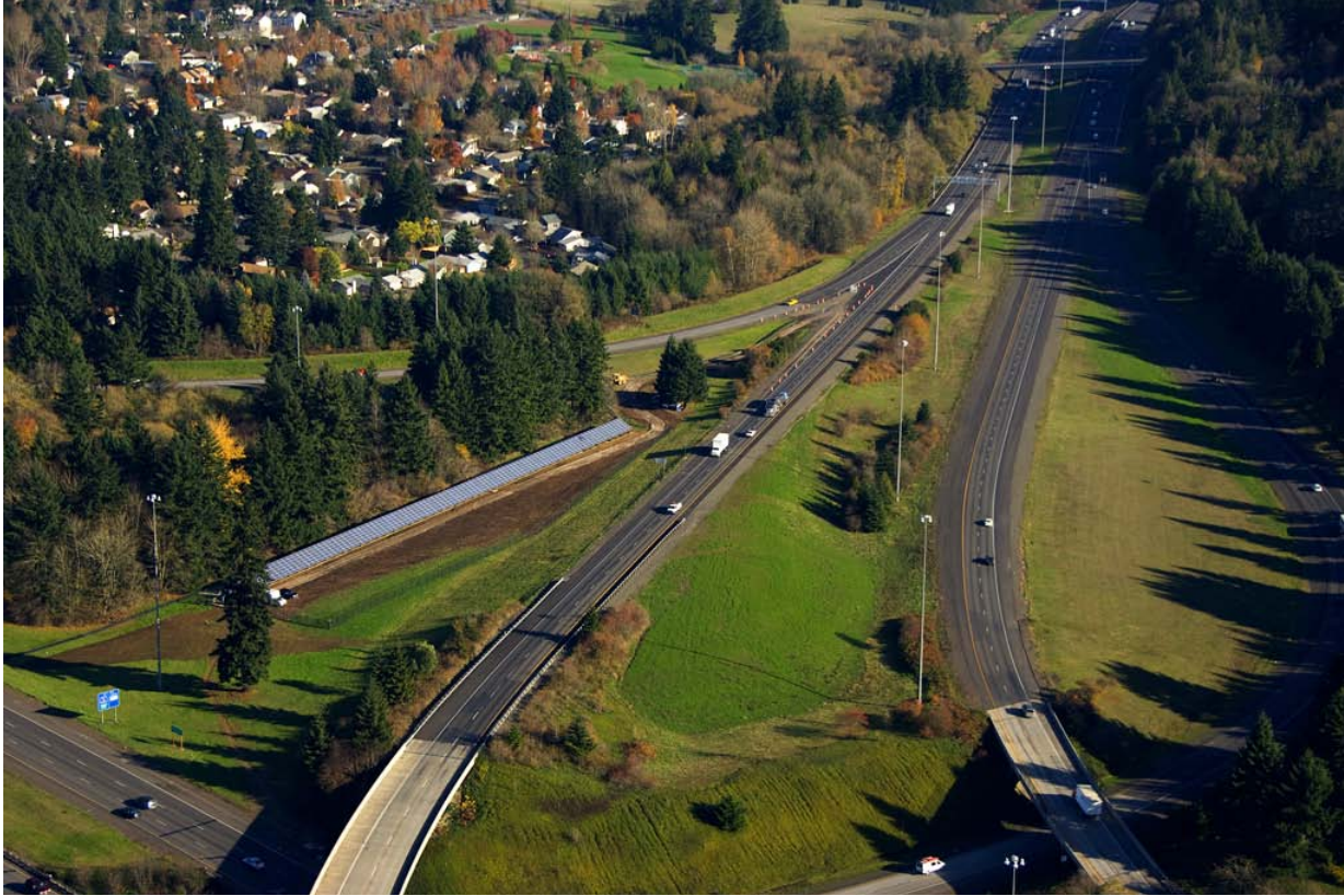
Figure 4 - Oregon Solar Highways project (Image: Oregon DOT)
