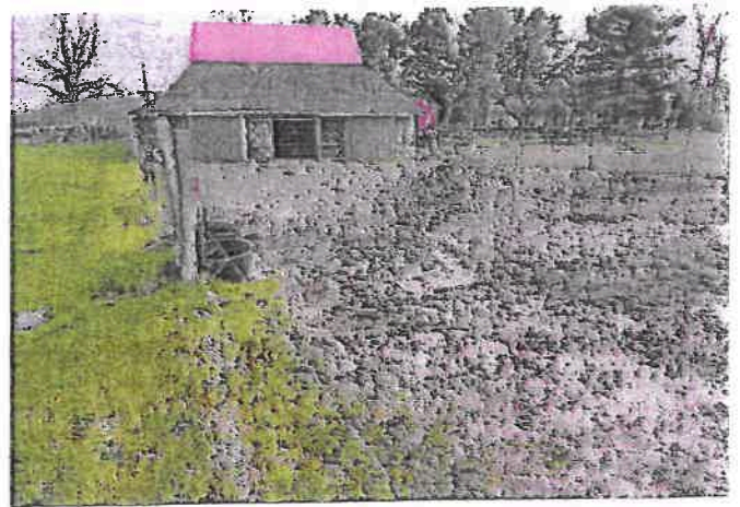
Photo 4: Poor condition electric fence along proposed TCA.
