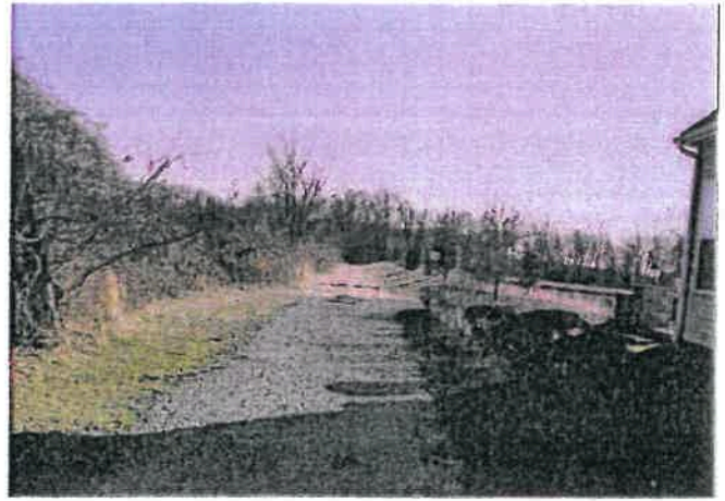
Photo 10: Existing stabilized access to proposed alternative looking toward sewer easement
