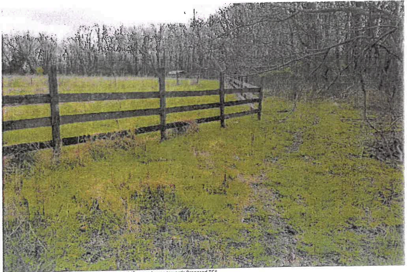
Photo 6: Existing sewer easement looking along the Wildflowers Access towards Proposed TCA.
