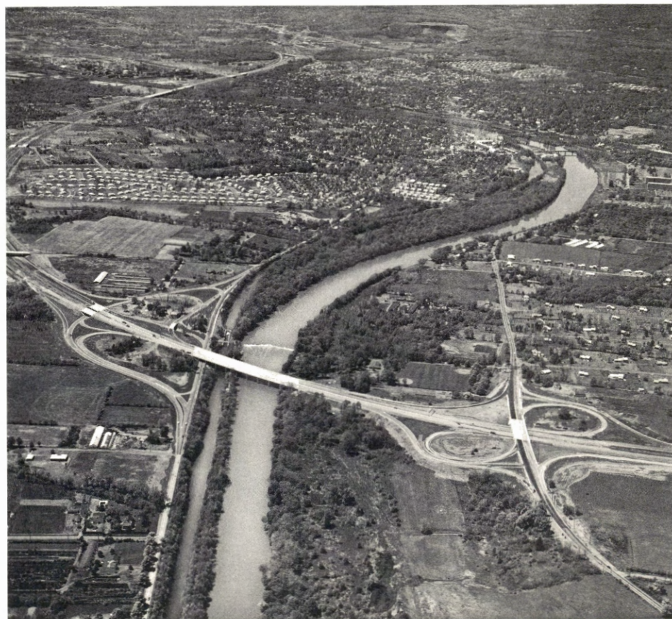
A COMPLETED MIDDLESEX EAST-WEST FREEWAY PORTION OF INTERSTATE ROUTE 287 IN THE BOUND BROOK AREA
