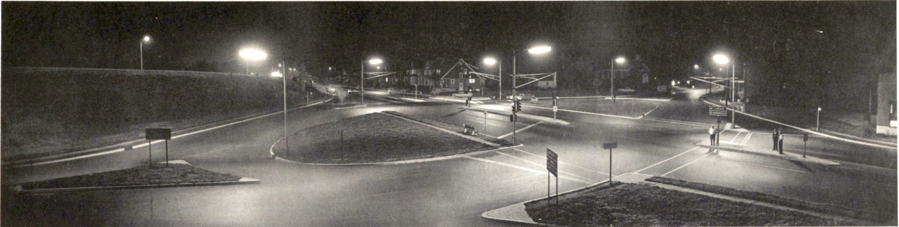
BLANKET LIGHTING OF CHANNELIZED INTERSECTIONS PROMOTES DRIVER SAFETY AND CONVENIENCE.
