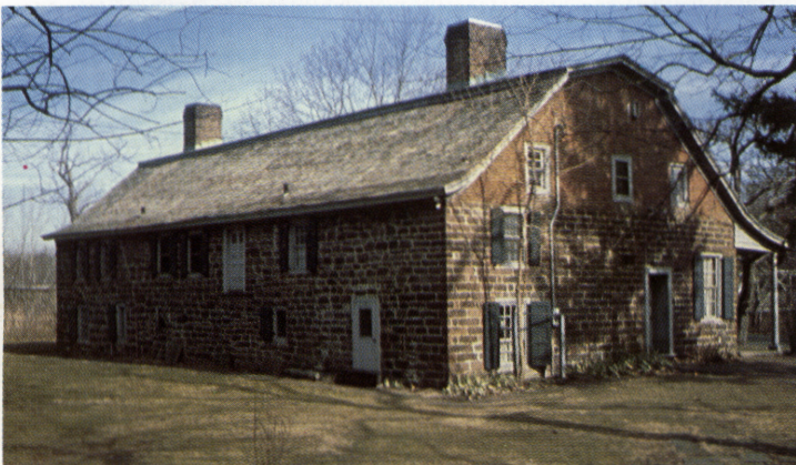
Von Steuben House, River Edge. Original section built 1737.
