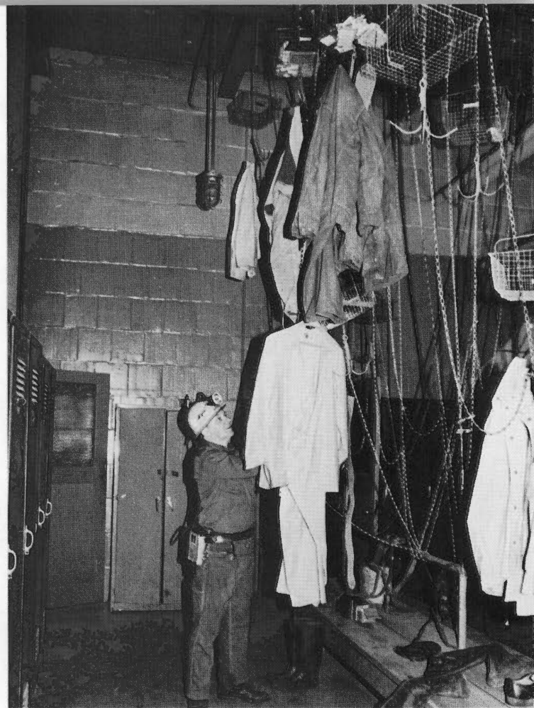
Shown hoisted to the ceiling in the “change room” are some of the open baskets used by miners for storage of their wet mine clothes where fans helped blow clothes dry before another day’s work in the tunnels below.
