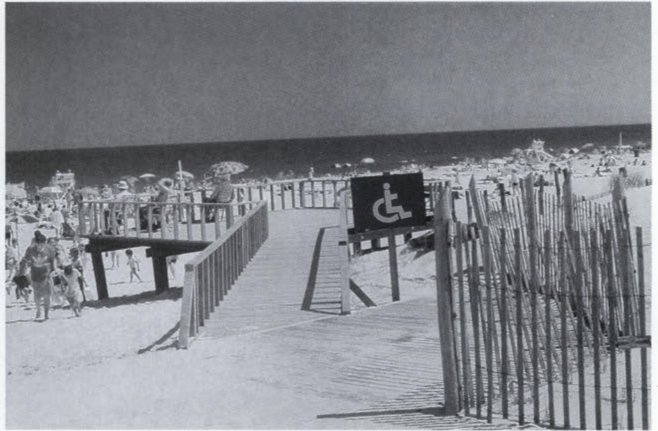
The barrier free ramp and deck at Island Beach State Park
