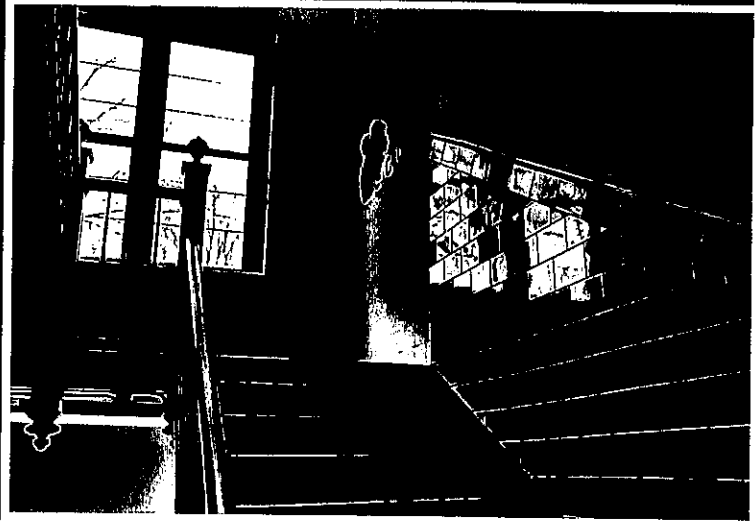
The only stairway leading to the busy lunch serving hall has just one hand rail.
