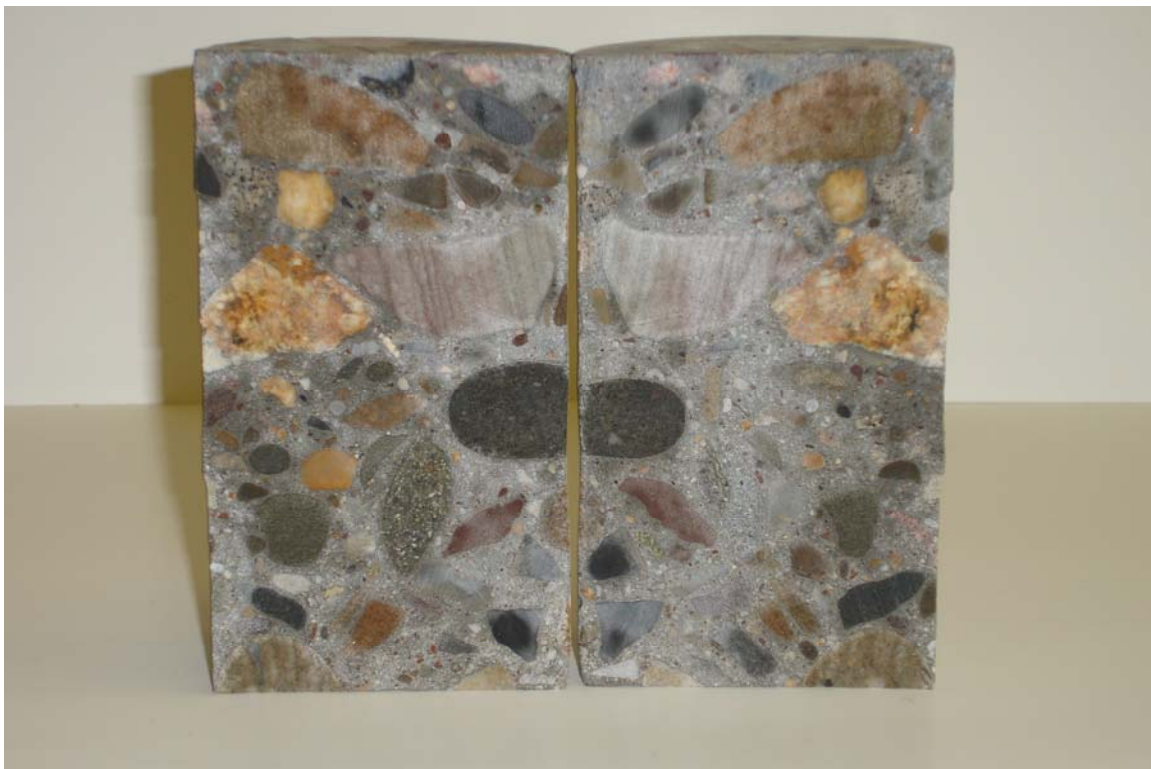
Figure 48 – Cross Sectional View of PCC Core Taken from Rt 202S in New Jersey
