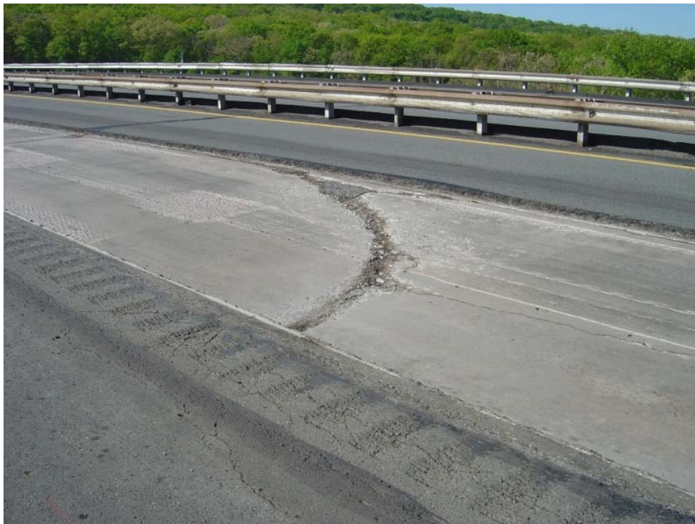
Figure 61 – Exposed Surface of Underlying PCC Pavement on Interstate 476 in Pennsylvania
