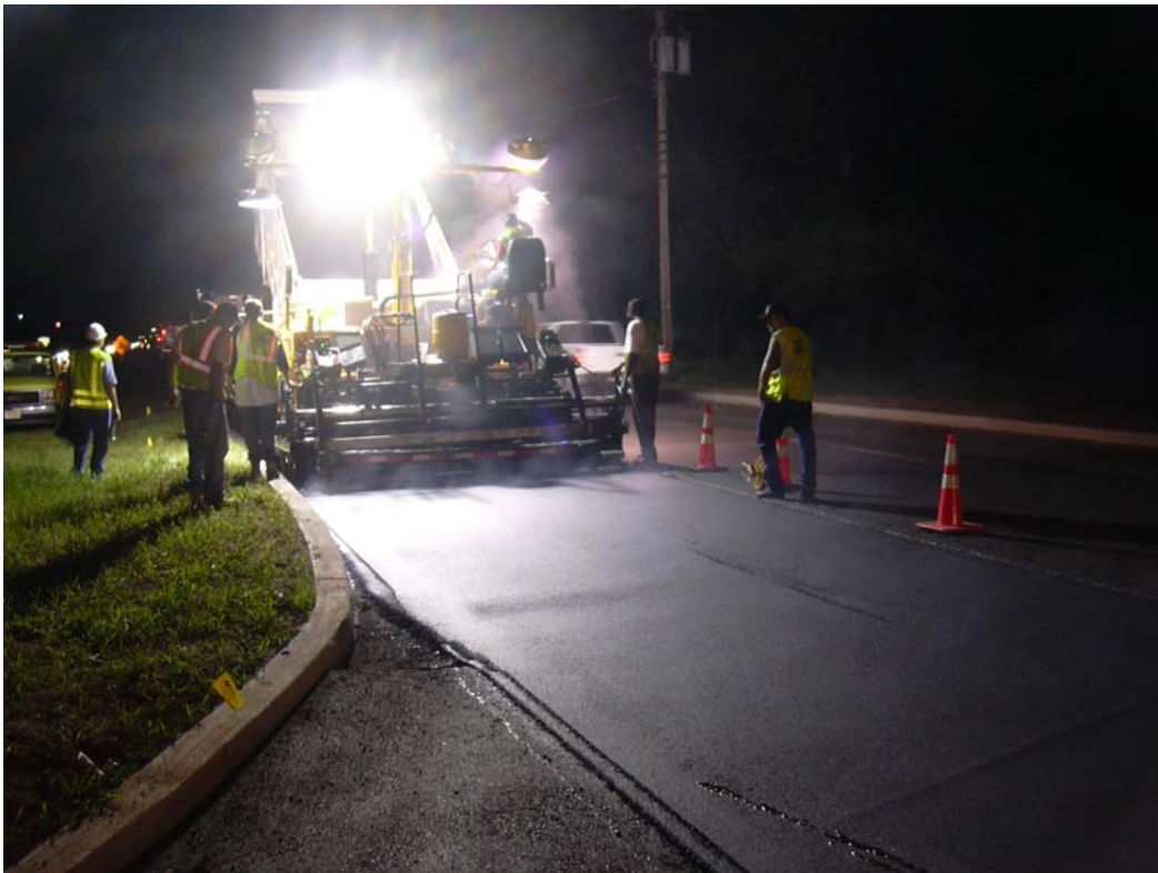
Figure 28 – Paving RCRI Mixture on Rt 34N in New Jersey
