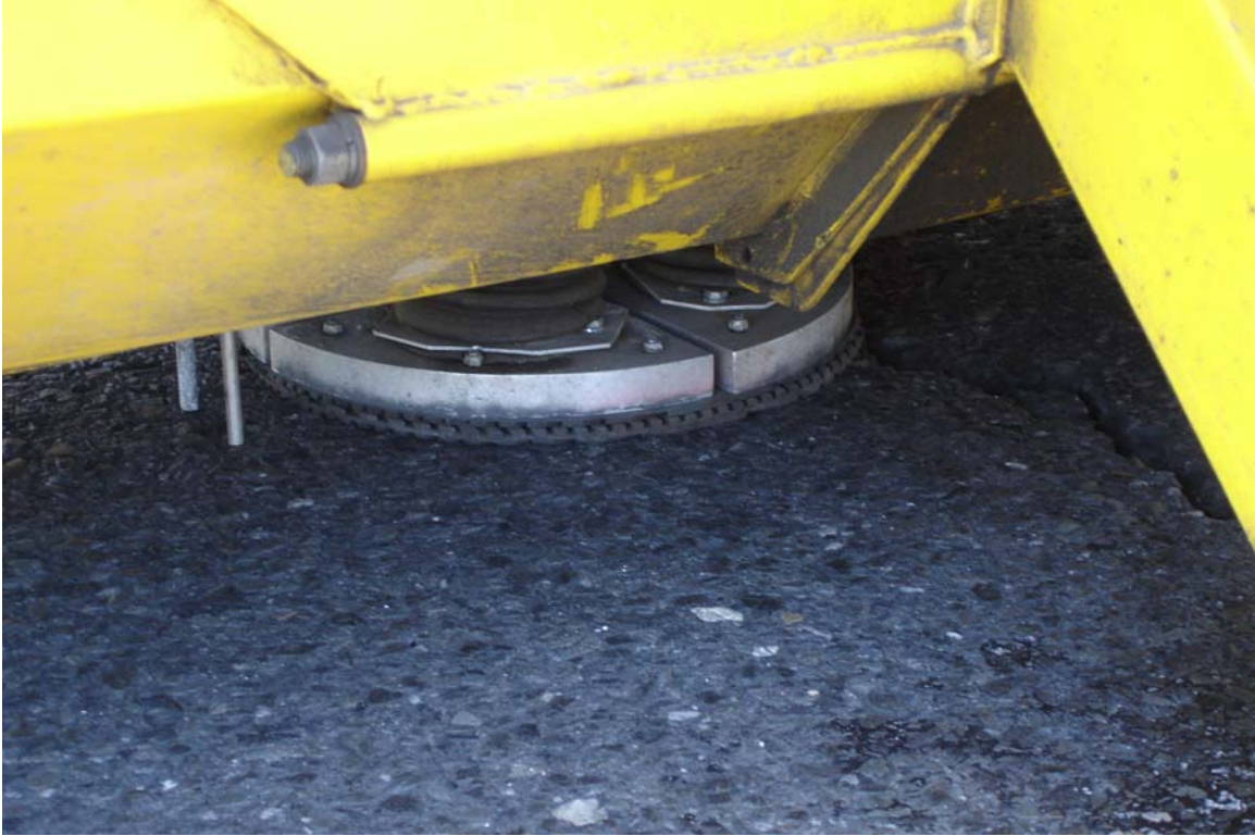
Figure 20 – Falling Weight Deflectometer (FWD) Testing at the PCC Joint
