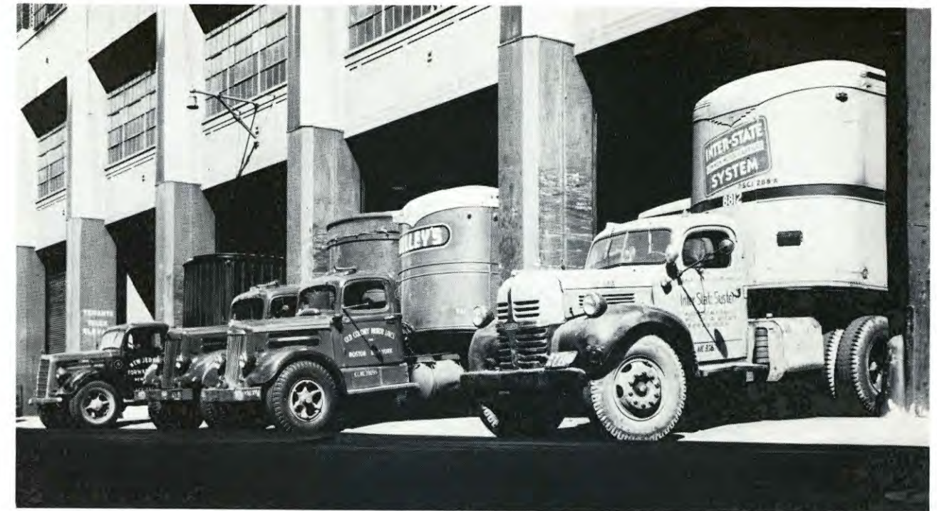
Street and basement floors of the Port Authority Building are occupied by the Union Railroad Freight Terminal
