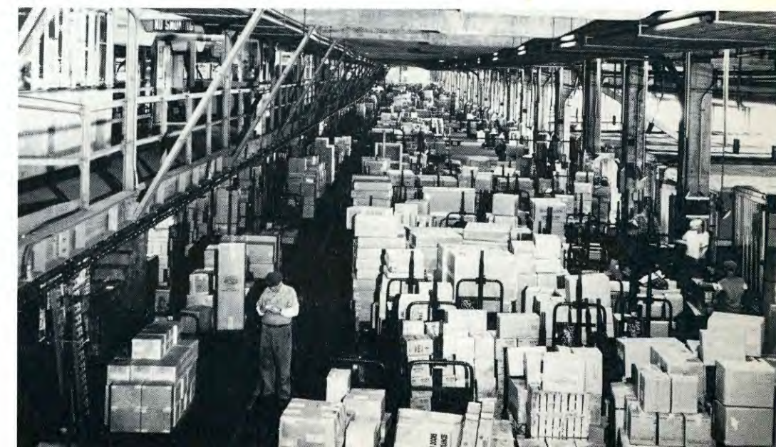
Business was brisk at the New York Union Motor Truck Terminal, with 1,000 tons a day handled across the platform during the peak season. Located near the Holland Tunnel and Manhattan's chief west side arteries, this facility helps reduce truck congestion in crowded city streets and helps speed terminal handling time for truck freight.
