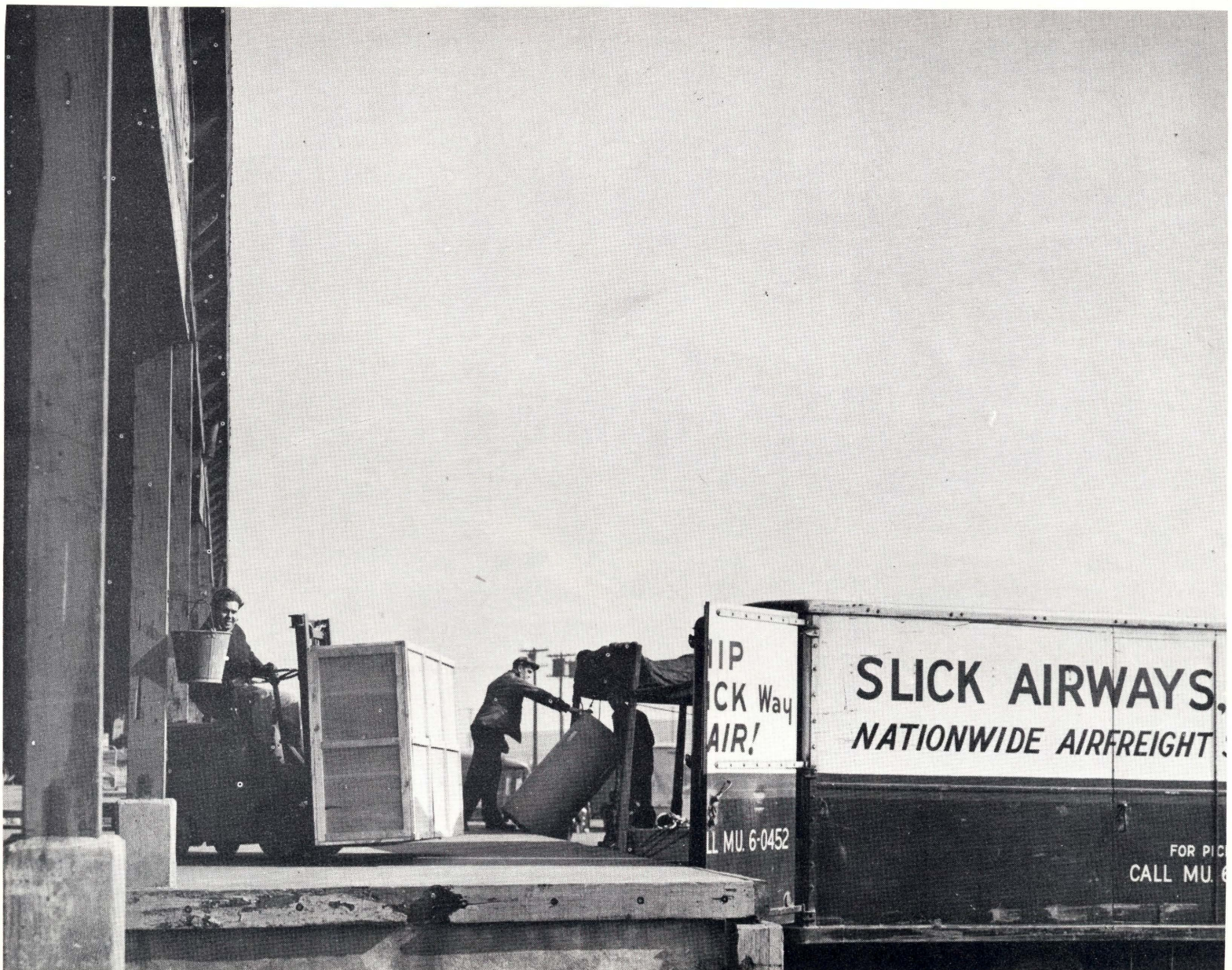
FREIGHT HANDLING AT THE BUILDING 50, AIR CARGO TERMINAL.
