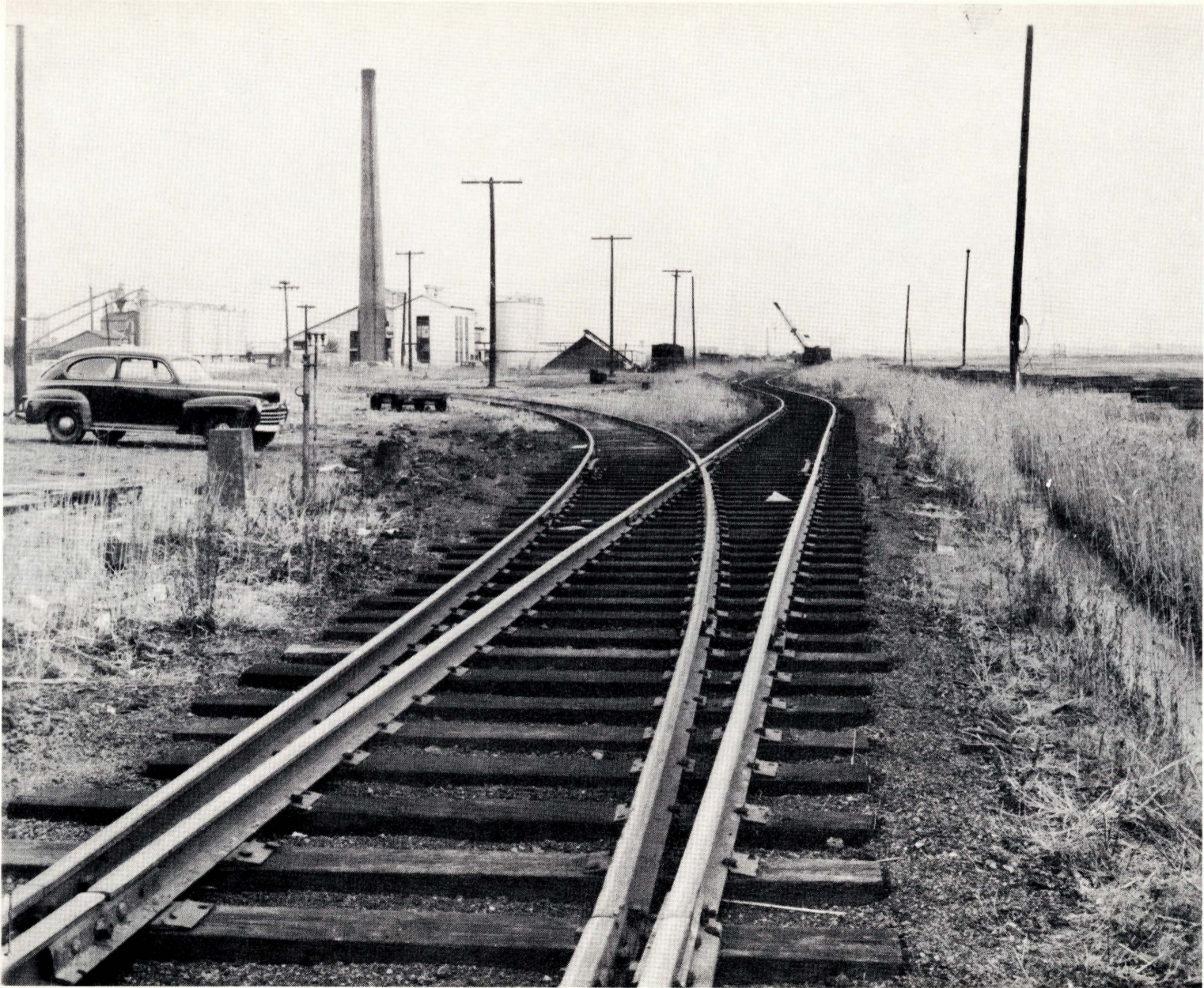
SECTION OF RAIL TRACK REHABILITATED BY THE PORT AUTHORITY, SHOWING NEW TREATED TIES AND NEW ROADBED.
