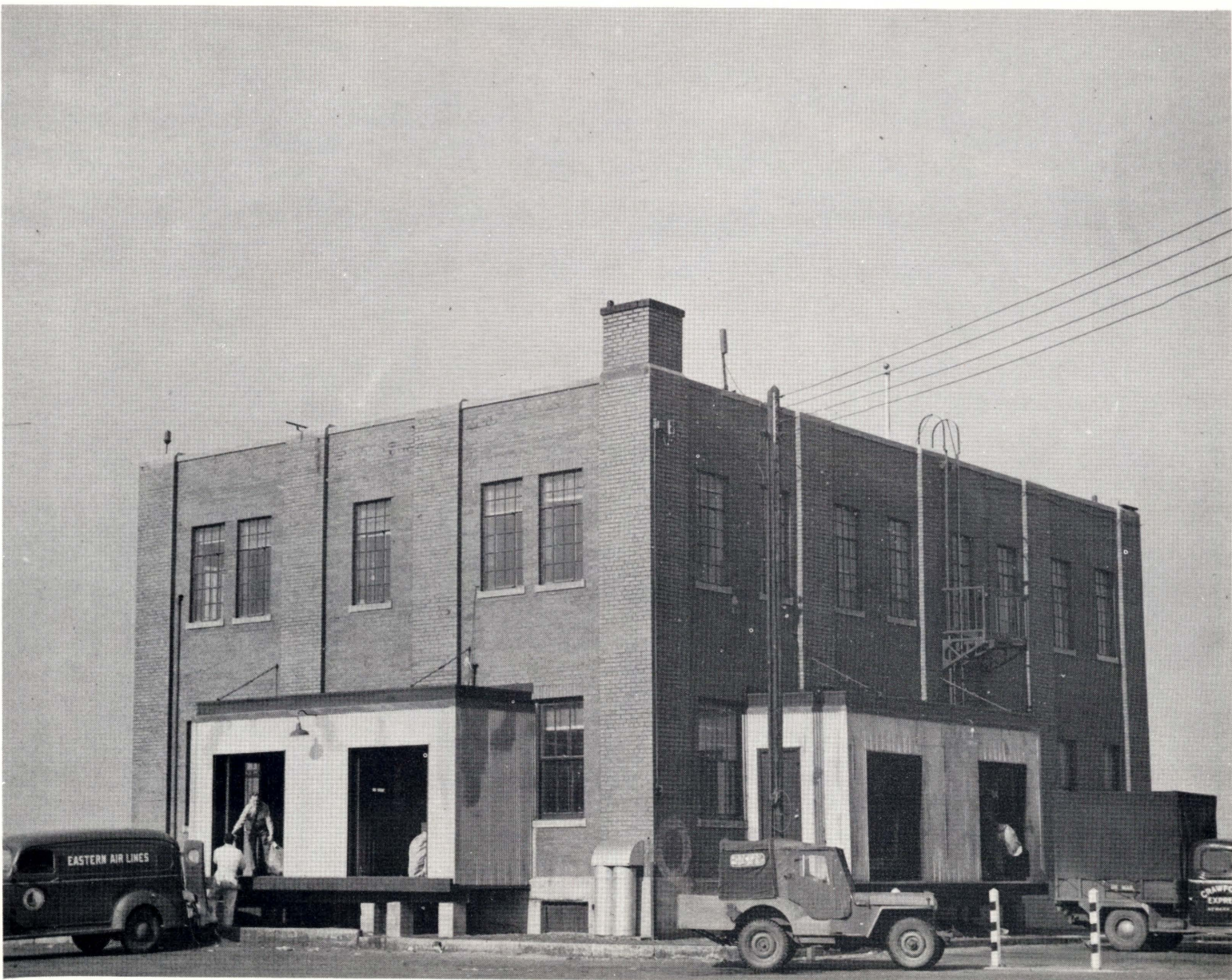
AIR MAIL FIELD OFFICE WITH TWO NEW EXTERIOR LOADING PLATFORMS.
