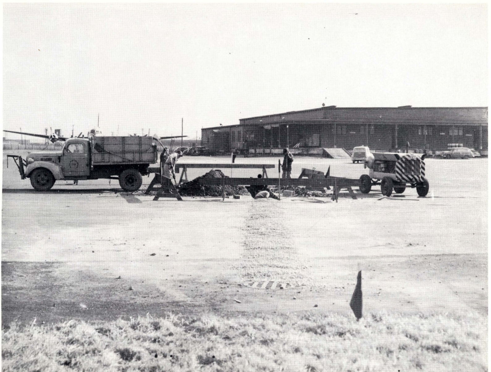
APRON DRAINAGE CONSTRUCTION NEAR BUILDING 50, AIR CARGO TERMINAL, KEEPS APRON CLEAR OF STANDING POOLS.
