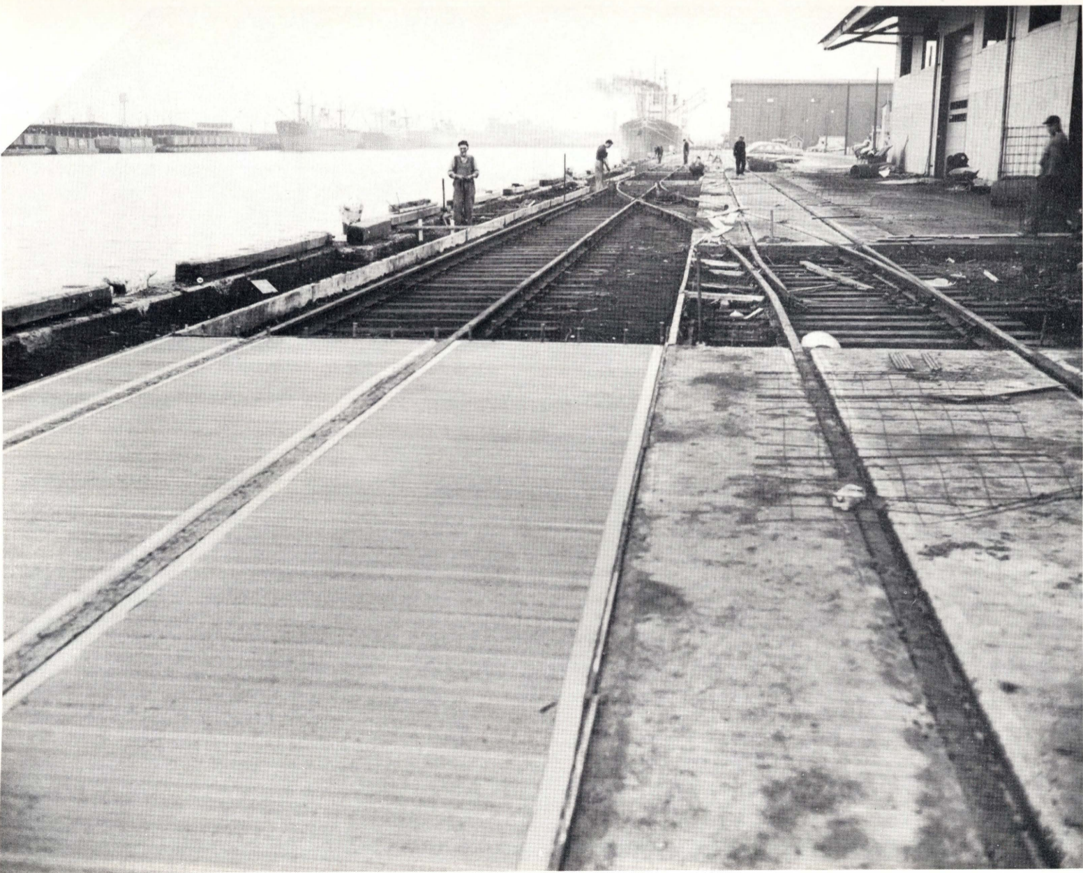
INSTALLATION OF NEW RAIL TRACKS AND PAVING IN FRONT OF THE NEW TRANSIT SHEDS.
