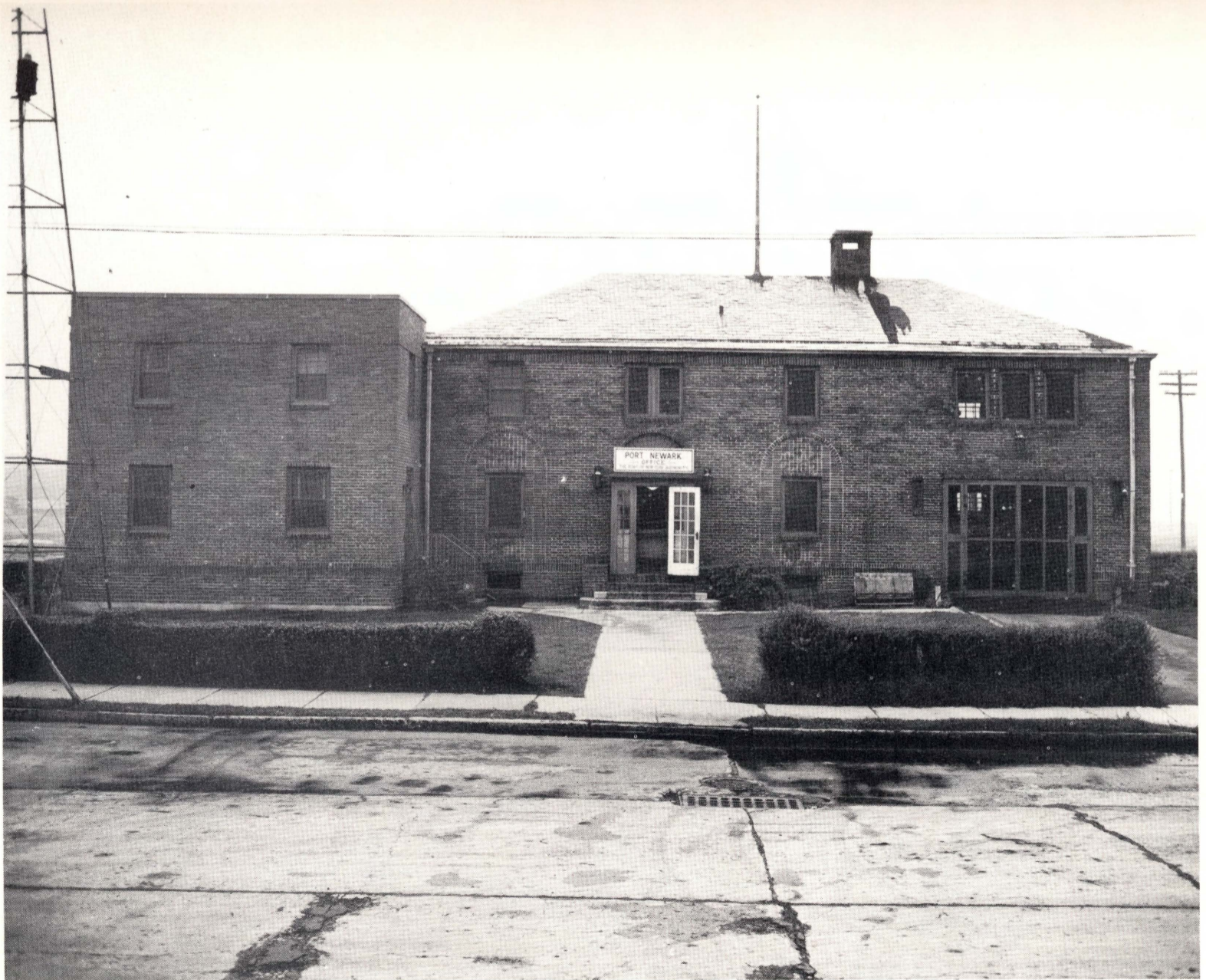
EXTENSION TO ADMINISTRATION BUILDING (SHOWN ON LEFT) BUILT BY PORT AUTHORITY TO HOUSE ITS PORT NEWARK OPERATING AND MAINTENANCE STAFF. QUARTERS FOR CITY OF NEWARK FIREBOAT CREW PROVIDED IN REMAINDER OF BUILDING.
