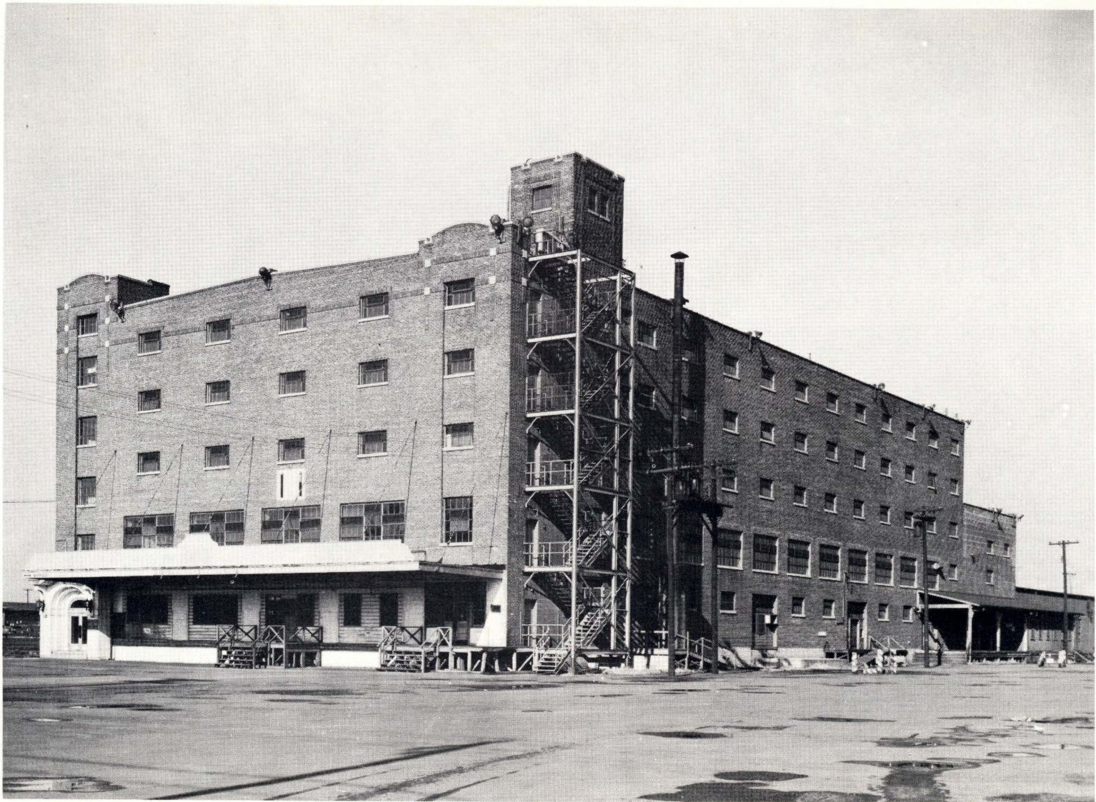
BUILDINGS 101 AND 101A WERE LEASED TO THE GARDEN SURPLUS SALES CORP. FOR PROCESSING AND DISTRIBUTION OF SALVAGE MERCHANDISE BROUGHT IN FROM OVERSEAS POINTS.
