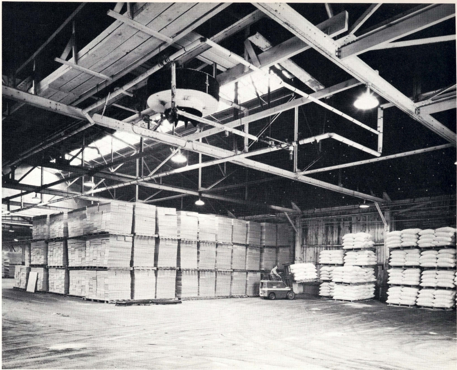
INSULATION BOARD, TAPIOCA AND STARCH STORED IN BUILDING 108 ON SOUTH SIDE OF PORT NEWARK CHANNEL.
