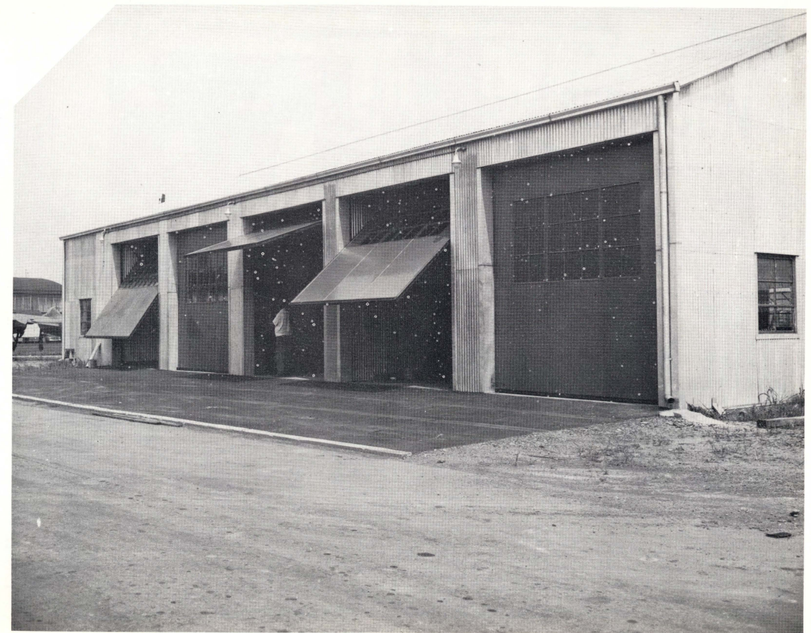
NEW EMERGENCY CREW BUILDING.
