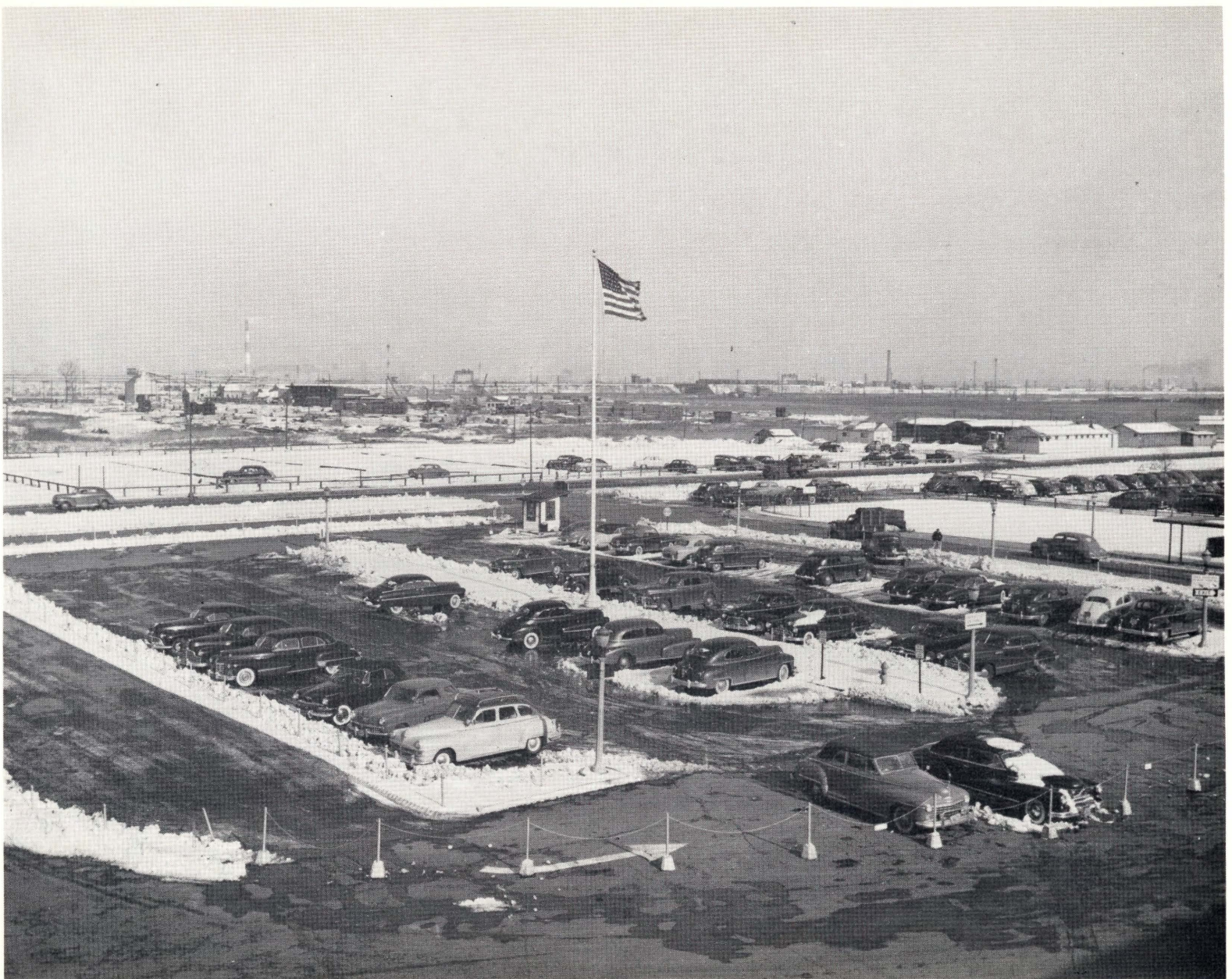
PARKING AREA IN FRONT OF THE TERMINAL.
