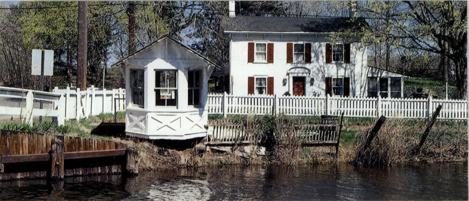
Canal, bridgetender's station and house in Blackswell's Mills
