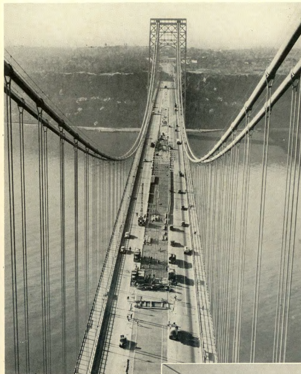
Above: With the paving of the two center lanes of the George Washington Bridge, eight roadways are now available to carry New York - New Jersey vehicular traffic over this great trans-Hudson span.
