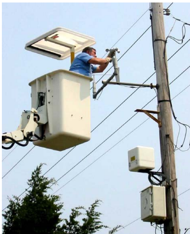
Figure 4: Servicing a CREST Monitoring Station
