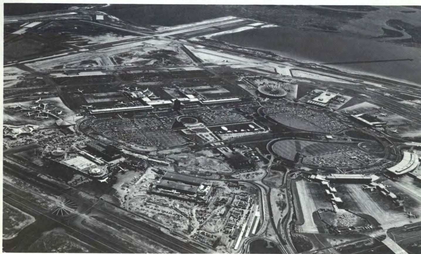
Port Authority expansion of the International Arrivals Building and the construction of additional terminals by the airlines are part of a $350 million construction program at Kennedy International Airport to keep pace with the demands of increasing volumes of air passengers.
