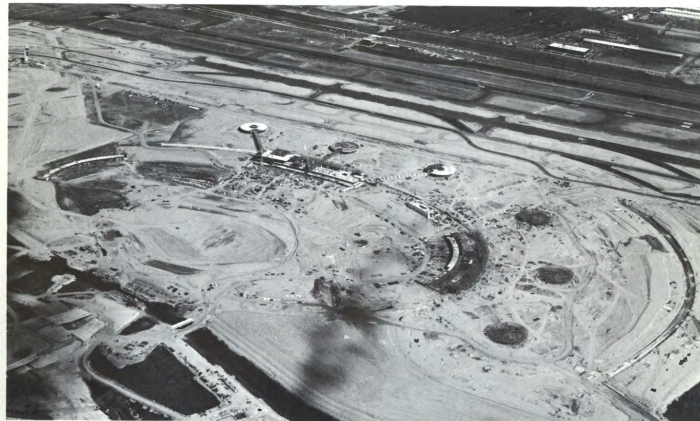
The $200 million redevelopment program in the Central Terminal Area at Newark Airport, comprising two terminal buildings and their six satellites, plus roadway and parking areas, was well under way in 1969.
