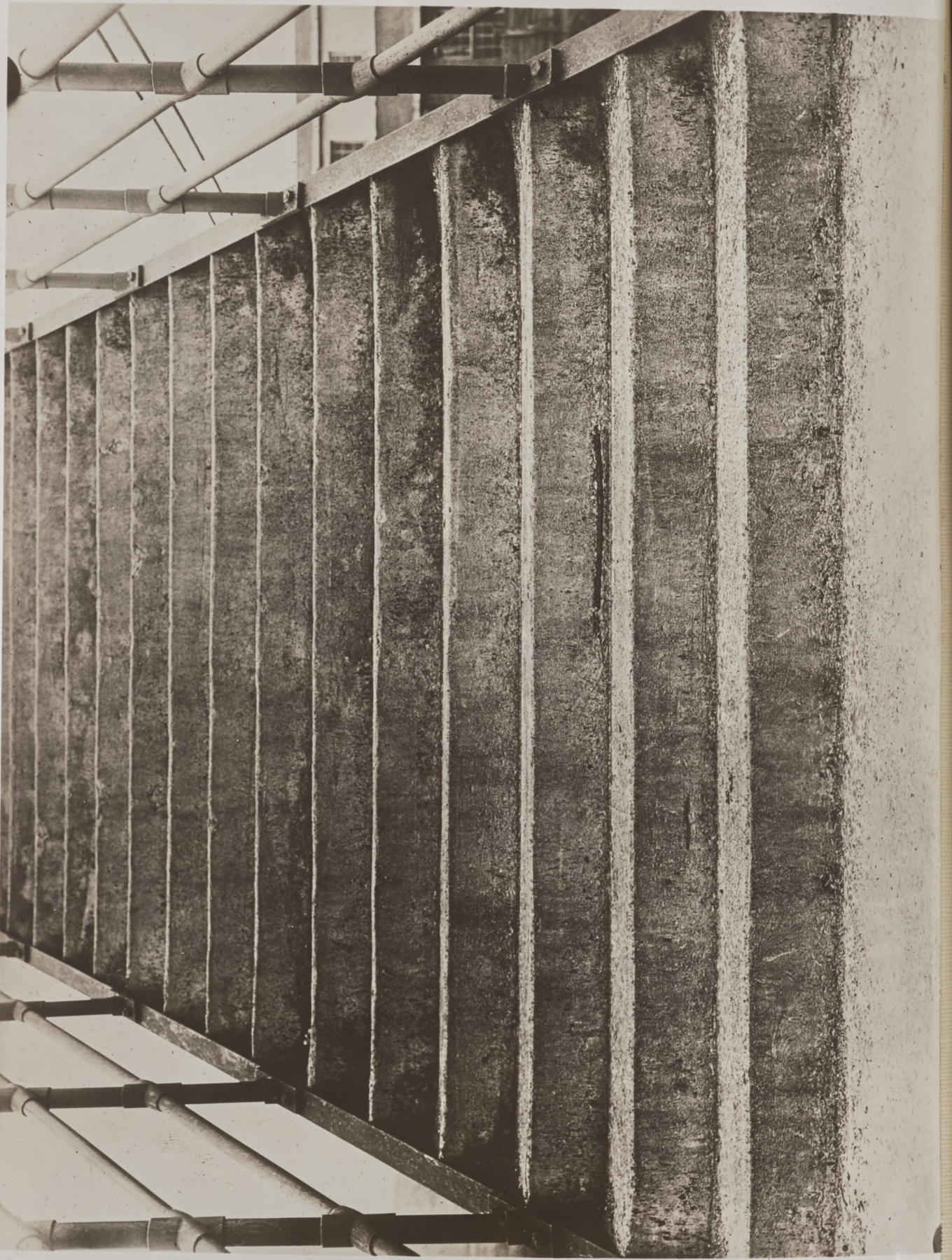
Lower Flight of Stairs of Westerly Approach.
